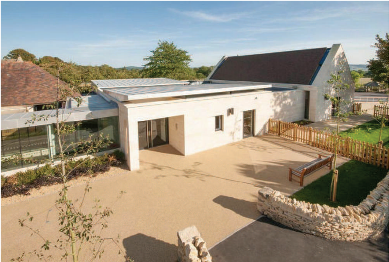
Overbury First School
