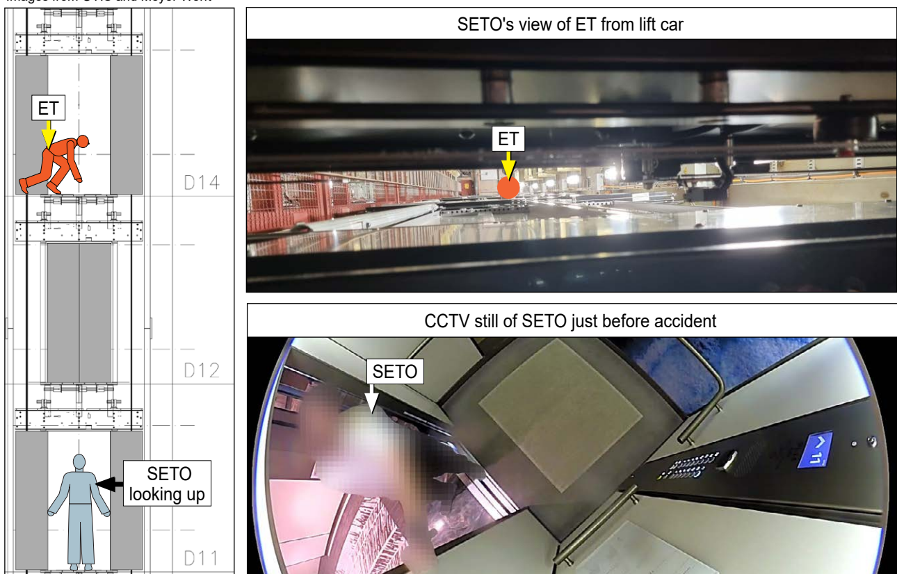
Figure 3: View looking up lift shaft from lift car
