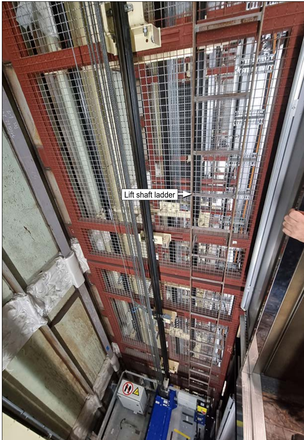
Figure 6: Lift shaft ladder viewed from deck 14
