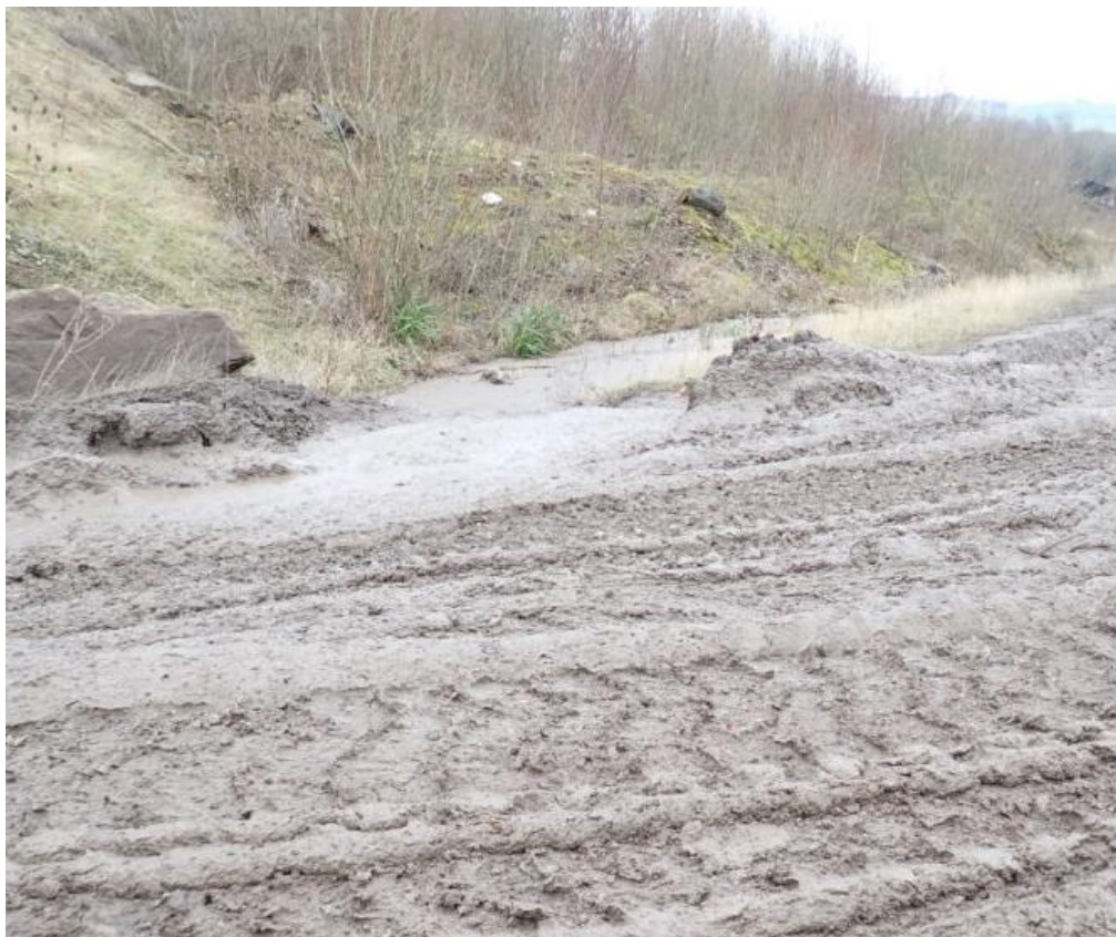
(Photos 12 - showing breach where mud and debris had flowed into the sites surface water management system)
