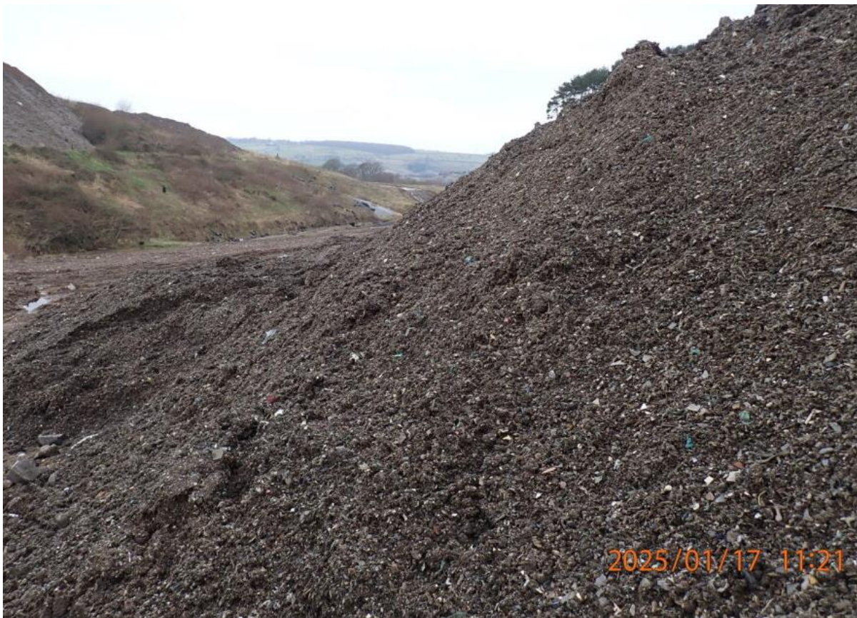
Photo 7 – waste fines situated in the centre of cell 5a
