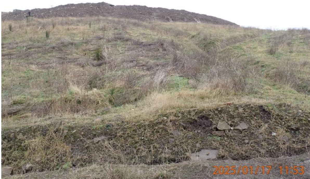
(Photo – 11 showing deposit of waste, believed to have been removed from the landfill, deposited on top of a previously capped area)
