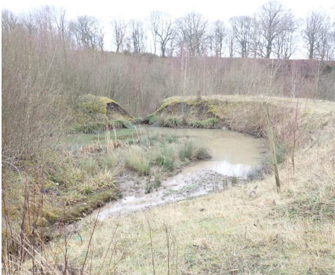
(Photo 10 - showing the first surface water management lagoon situated outside of the permitted area)
