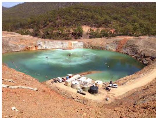
Figure 3: Virtual curtain treatment of contaminated wastewater in pit [Image Credit: CSIRO] [16].
