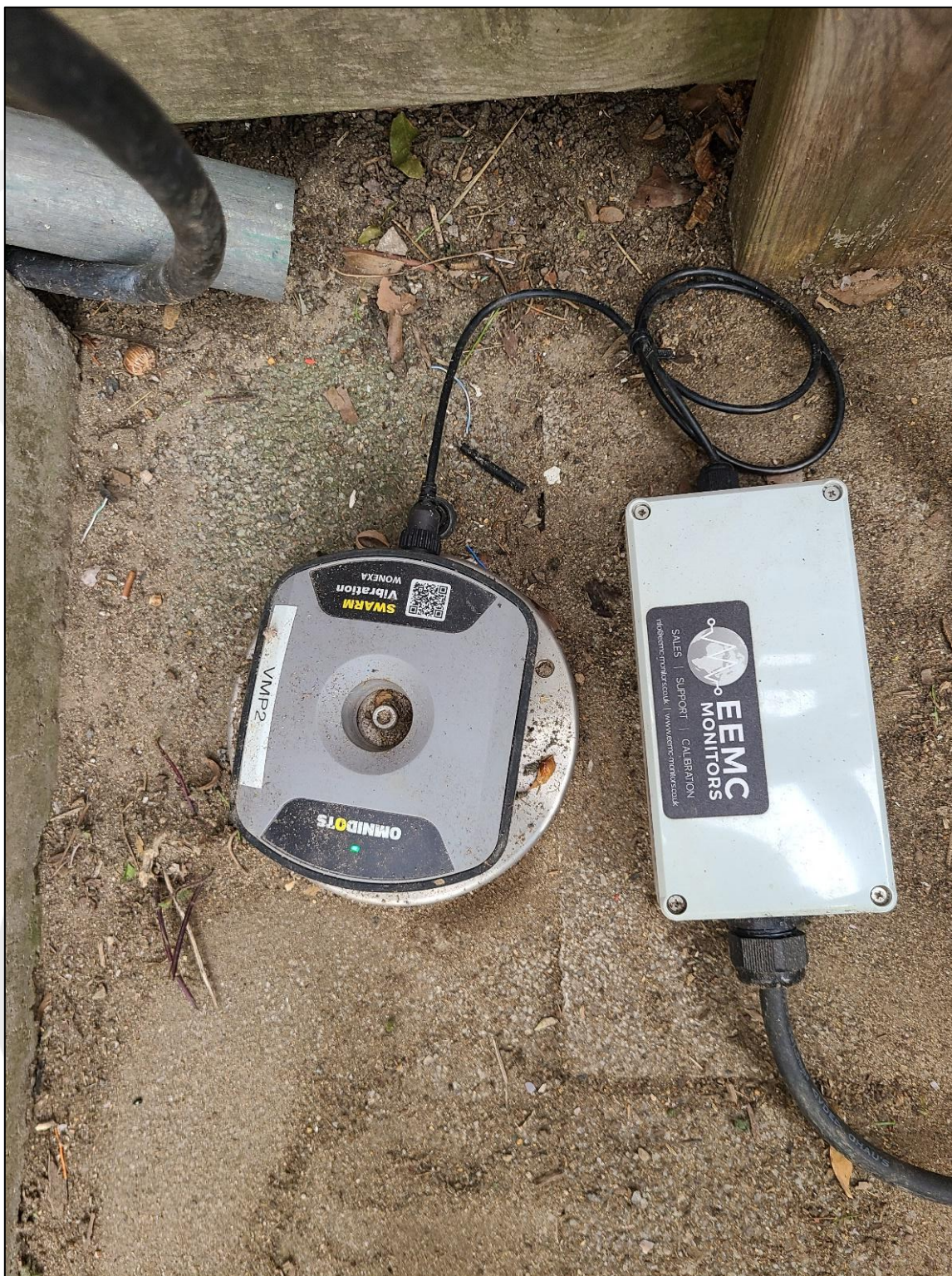
Image 2 –VMP2 Monitoring Location
