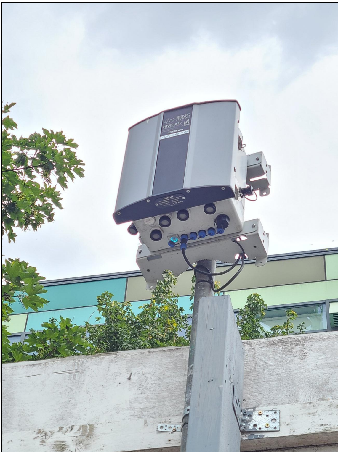
Image 2 – DMP2 Monitoring Location (photo taken on site on 24/07/2026).
