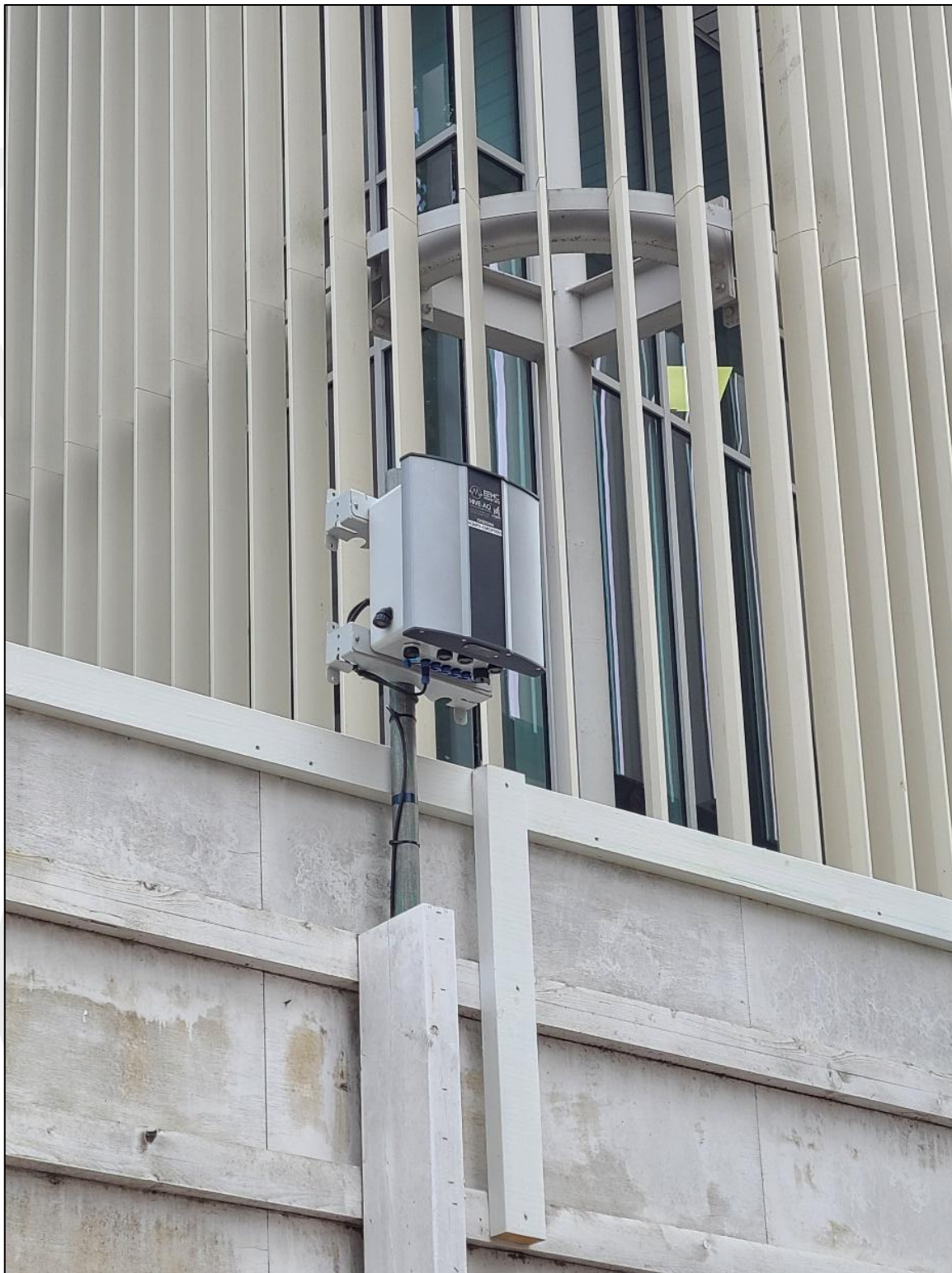
Image 3 – DMP3 Monitoring Location (photo taken on site on 19/5/2025).
