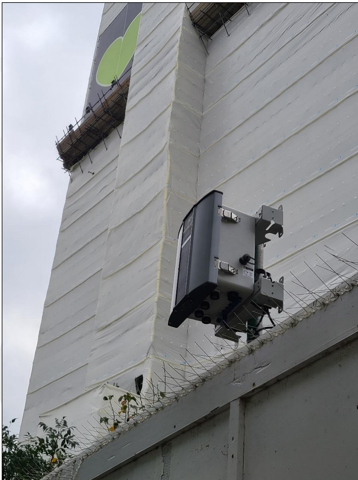
Image 1 – DMP1 Monitoring Location ( photo taken on site on 19/5/2025 ).
