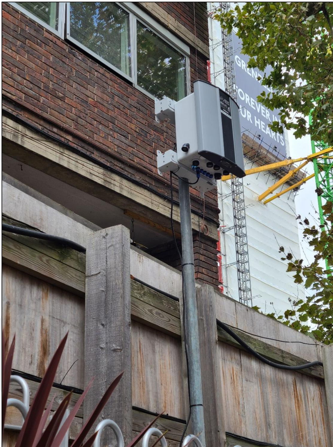
Image 4- DMP4 Monitoring Location (photo taken on site on 19/5/2025)
