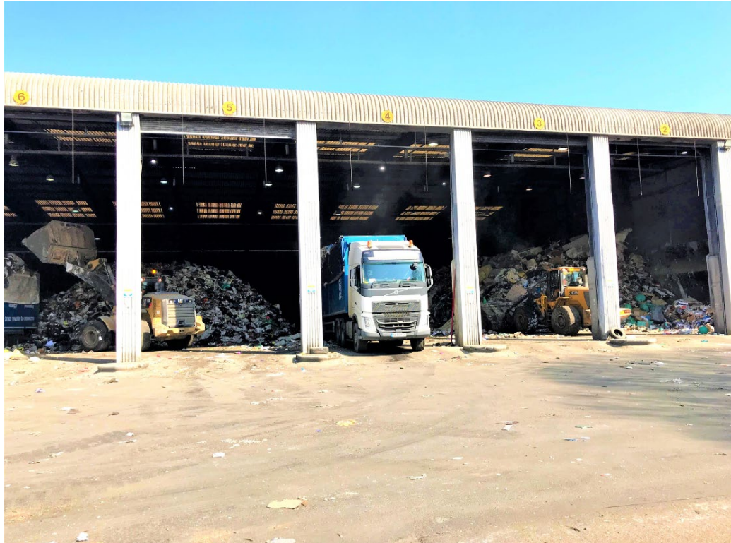
Figure 4. Residual waste tipping hall at Waterdale Waste Transfer Station
