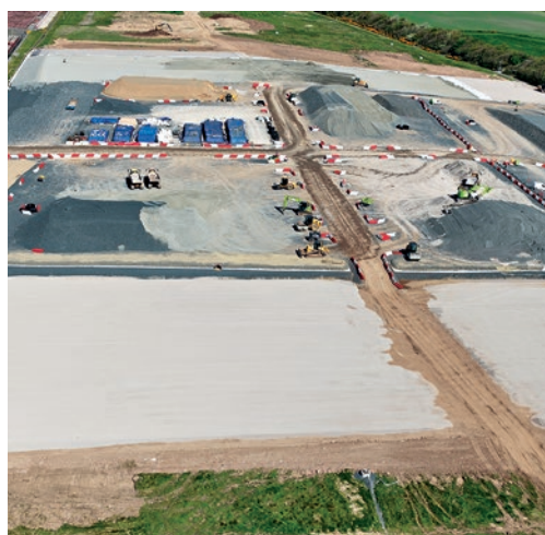
An aerial view of the trench cap
