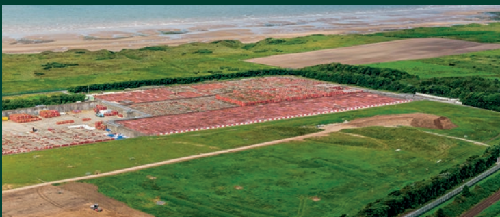
VOCD will include capping Vault 8 and the northern trenches
