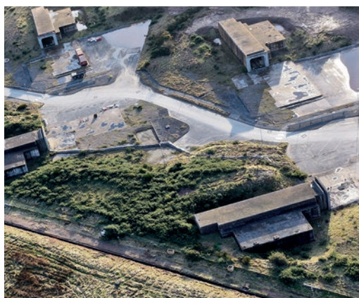
The demolition of the magazines is key for our capping operations
