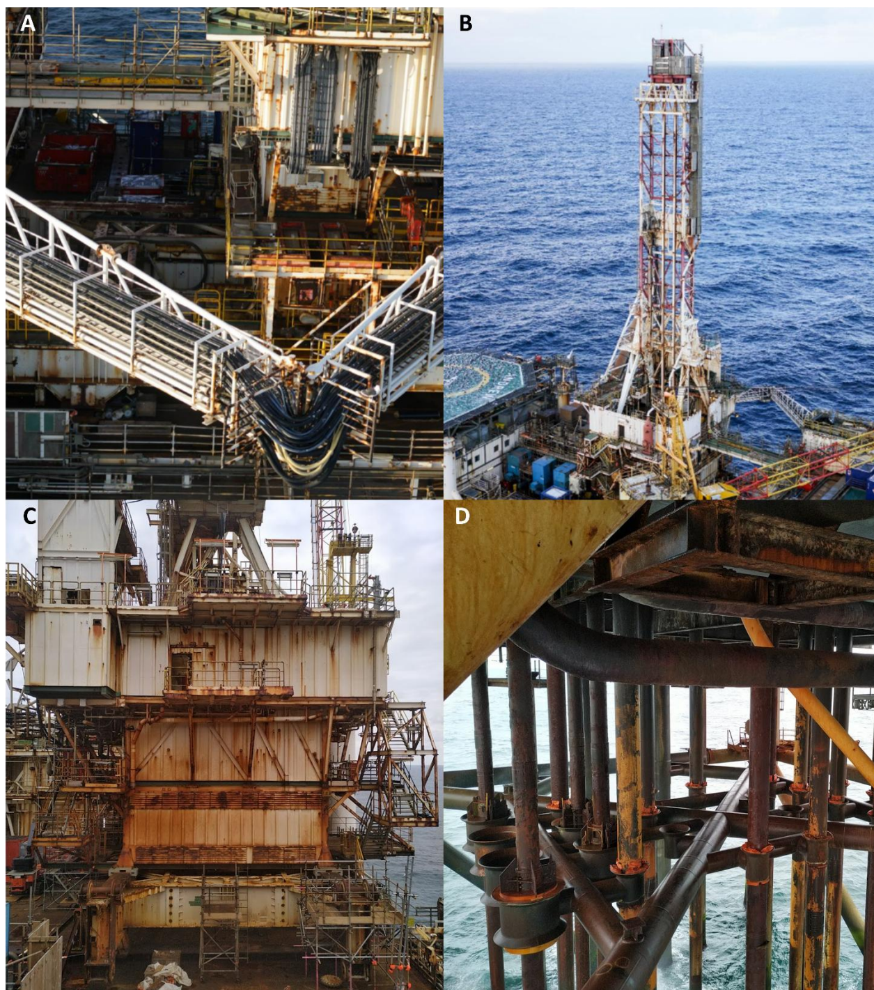
Figure 4-14: Drone photos of the articulate arm (A), DES (B), the decks (C) and the substructure (D) prior to the removal of the articulated arm and DES.
