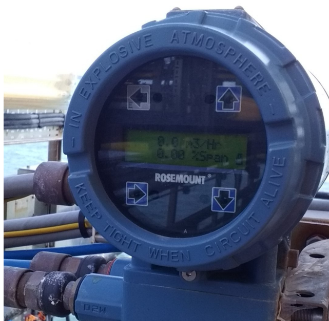
Figure 12: Coriolis meter to measure volumes of produced water re-injected
