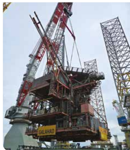
Galahad topside landed on grillage
