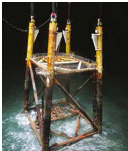
C1D jacket lifting operation
