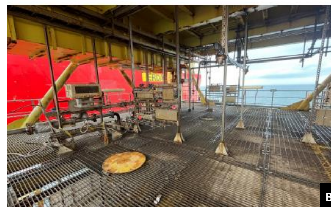
Figure 6: Well bay on the Wenlock installation (A) pre-P&A activities and (B) post-P&A activities.
