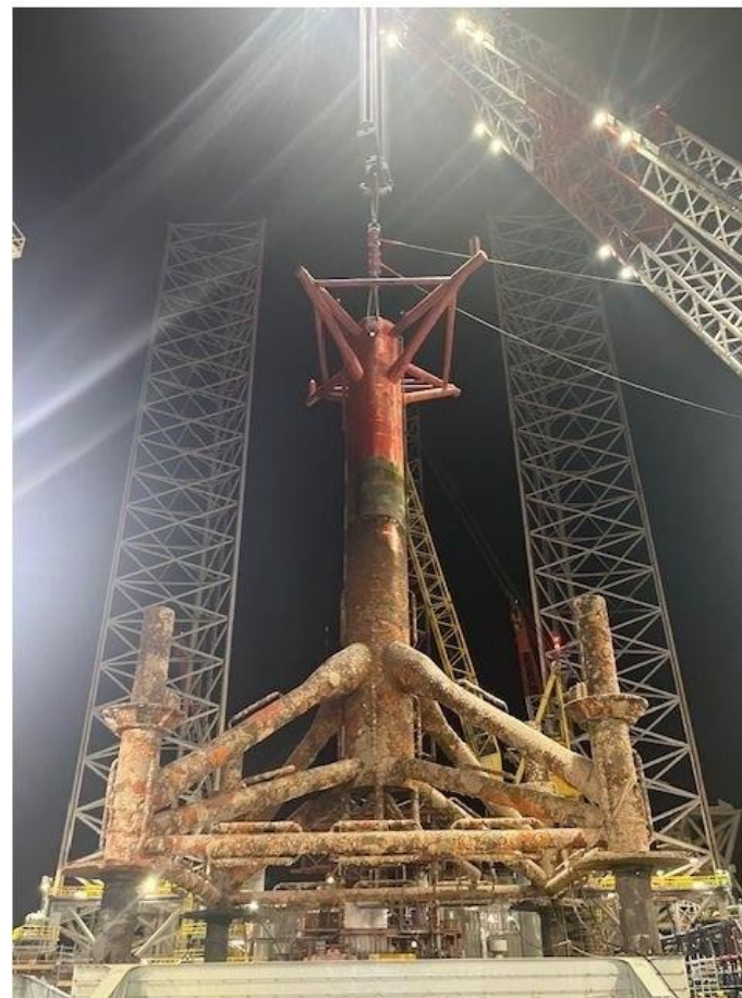
Figure 1: Removal of the Galahad monopod by the OBANA's 2,000 tonne crane.
