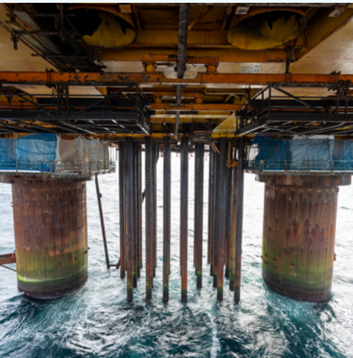
▲ Cormorant Alpha Well Conductors and Legs, showing leg cut working platforms
