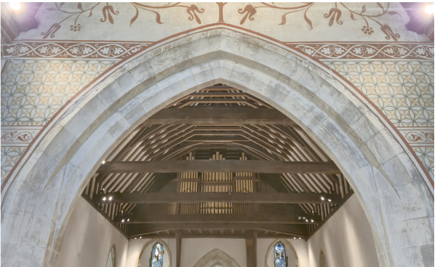
Image: Fluorescent lights were replaced with an energy-efficient LED system as a result of a successful CIP at St Peter's Preston Park © CCT
