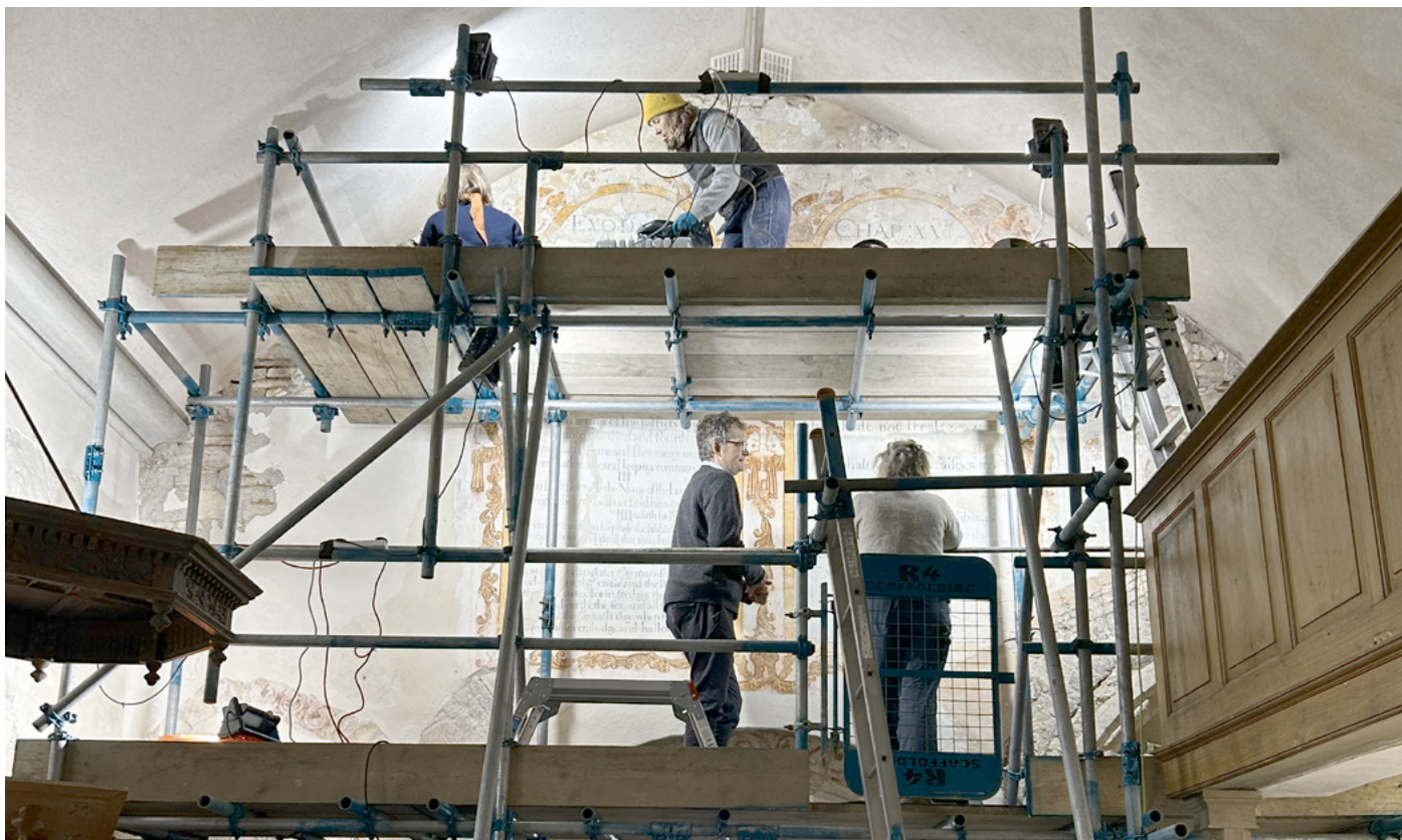
Conservation work in action at St James' Church, Cameley © CCT
