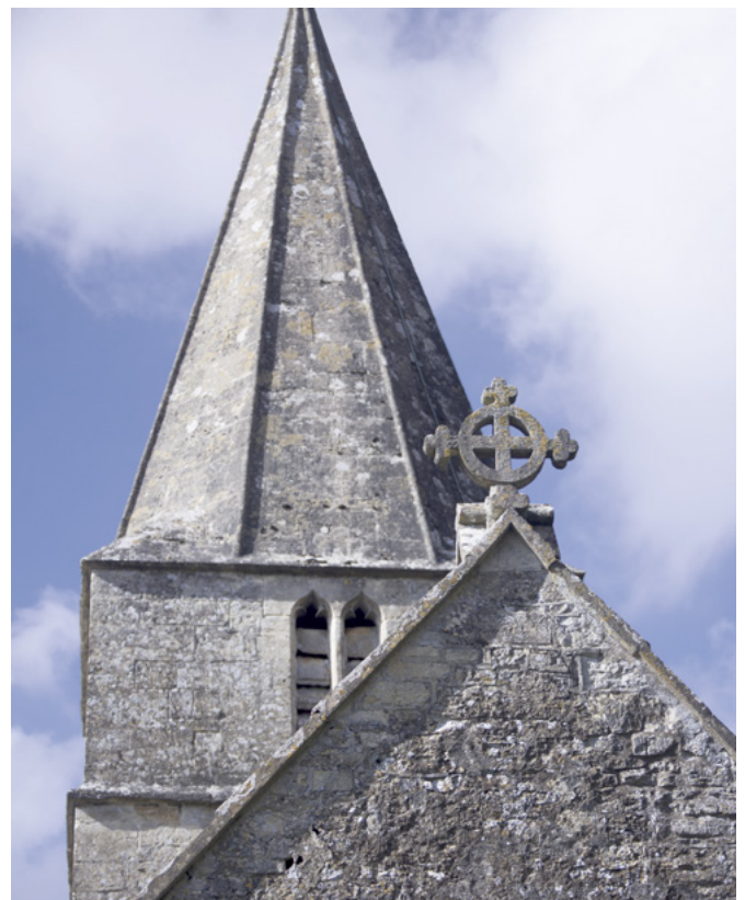
Image: The roof space at St Kenelm's Church is home to eight species of bats © Andy Marshall
