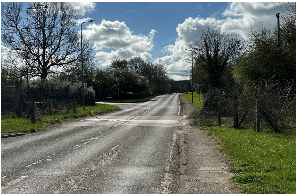
Photograph 3-2: B4011 Adjacent to the Southern Site Access
