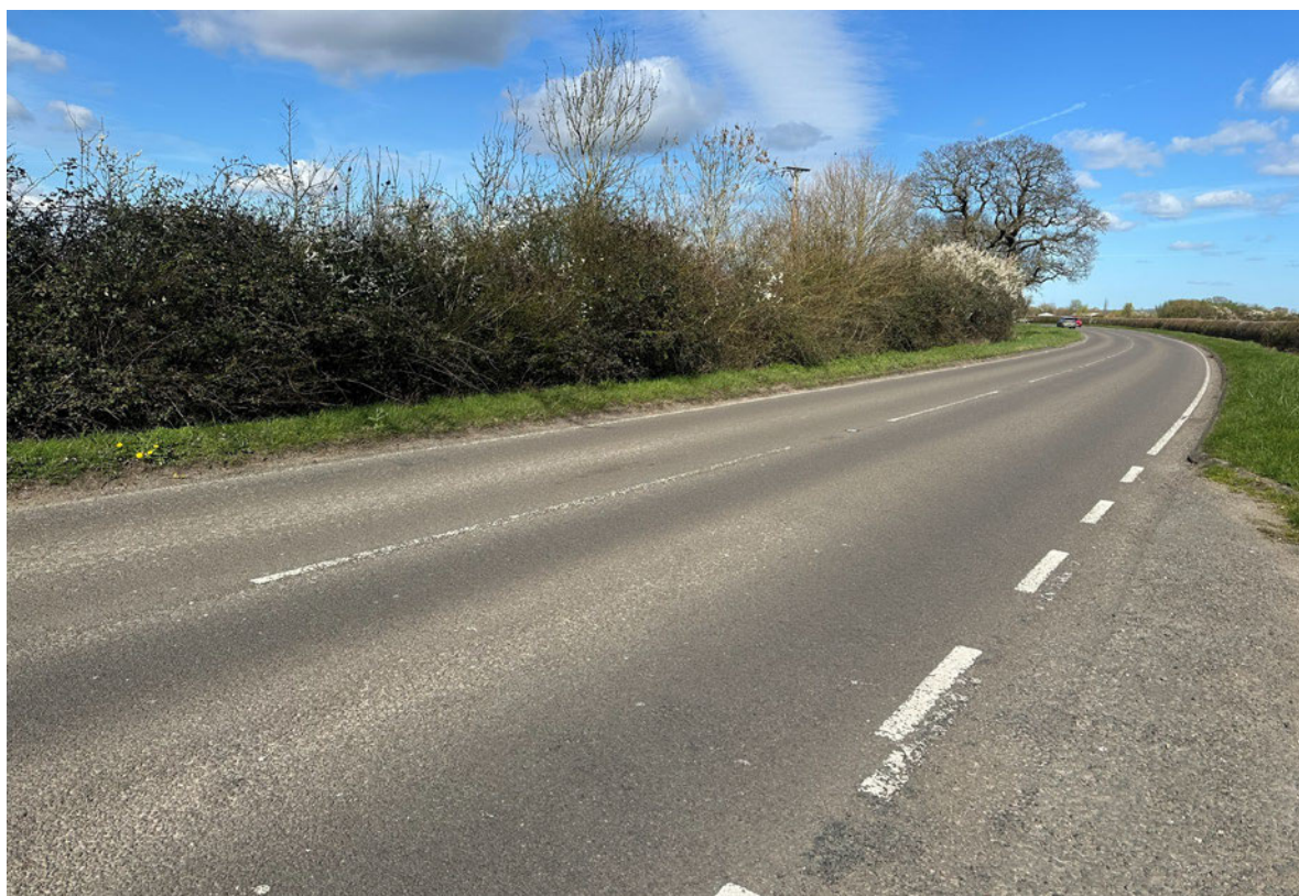
Photograph 3-1: B4011 Adjacent to the Northern Site Access
