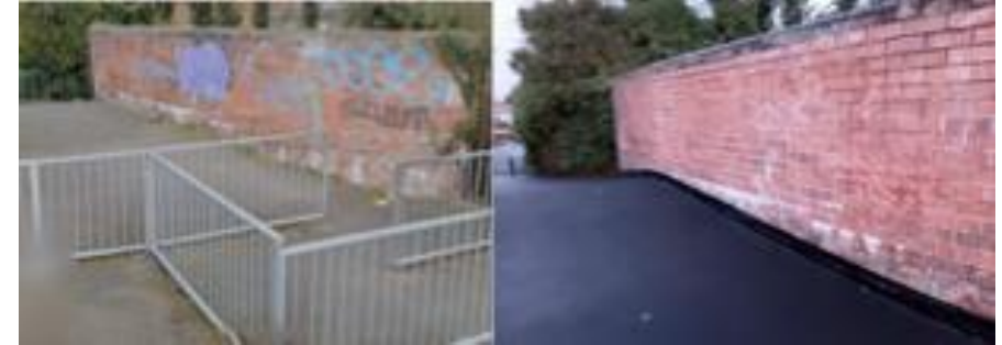
Bridge Repairs and resurfacing, Moathouse Lane, Wolverhampton
