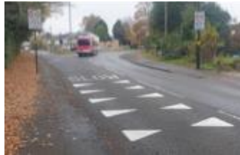
Hollyfield Road, Birmingham
