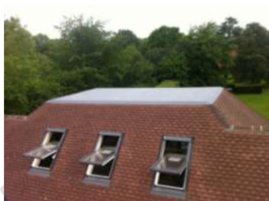
Figure 2.23: Example of a crown roof used to create additional habitable space in the roof.
