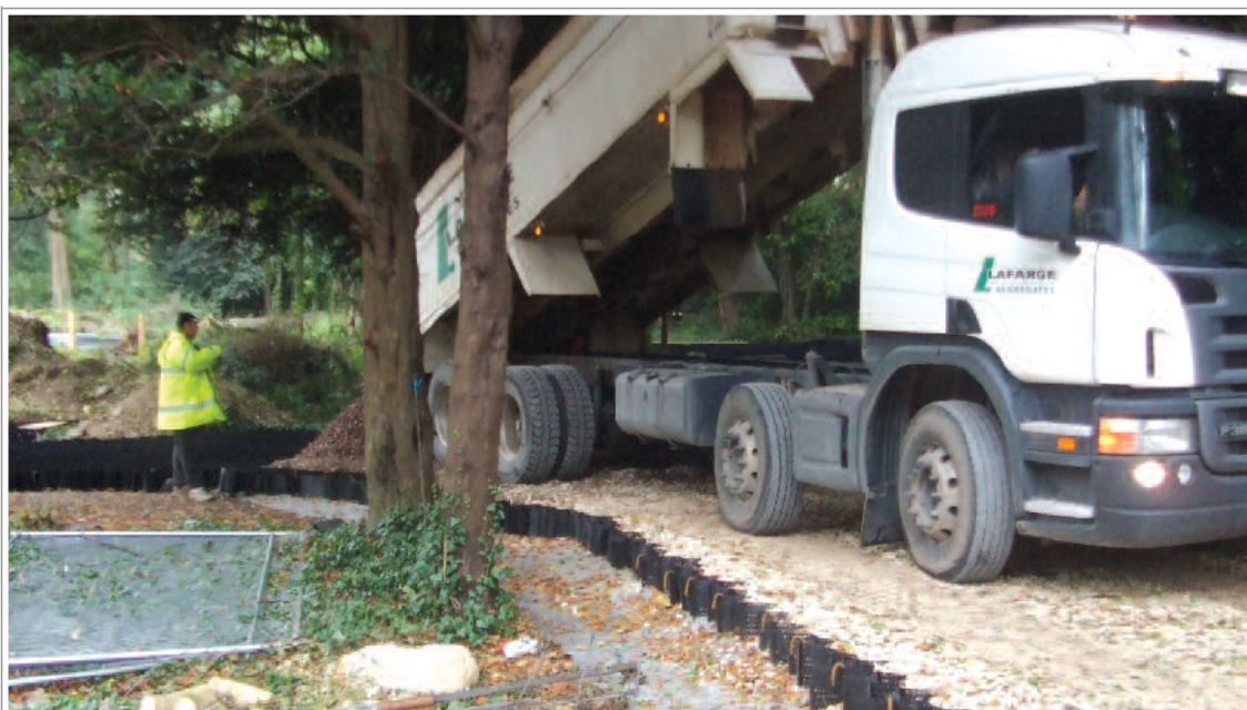
Installing a special surface to allow for heavy plant access through sensitive woodland during construction.
