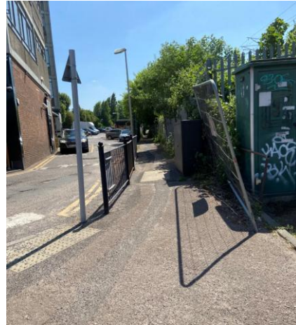
Photograph 16: Entrance to Segregated Footway at Darkes Lane
