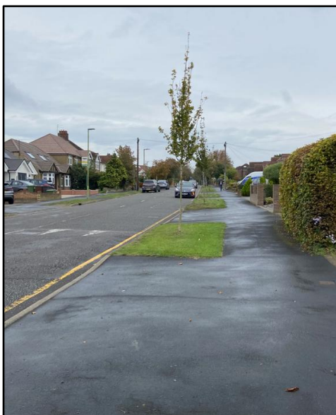
Photograph 9: Footway at The Walk
