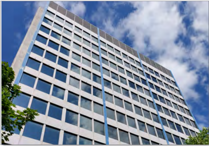
Building 2 - Maple House Eastern elevation. Photograph taken 16/06/2025.
