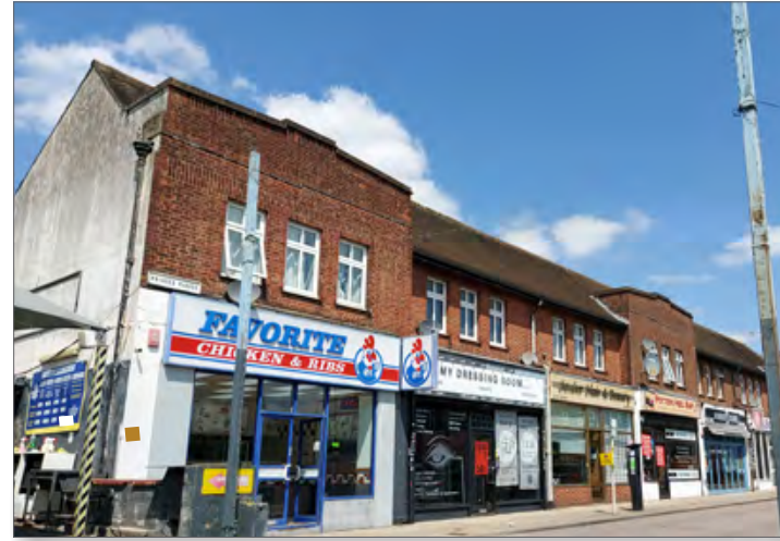
Building 8 - Princes parade Eastern and southern elevations. Photograph taken 16/06/2025.
