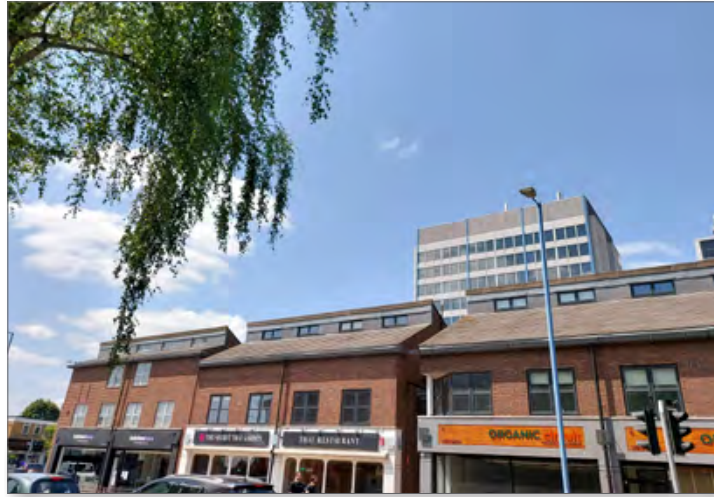
Buildings 3 to 7 - High Street Eastern elevation. Photograph taken 16/06/2025.
