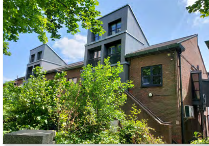
Buildings 3 to 7 - High Street Western and southern elevations. Photograph taken 16/06/2025.
