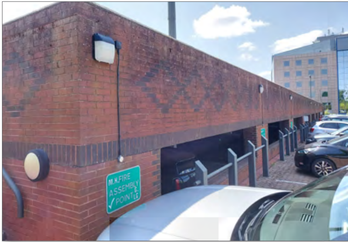
Building 9 - Parking Garage Western and southern elevations. Photograph taken 16/06/2025.
