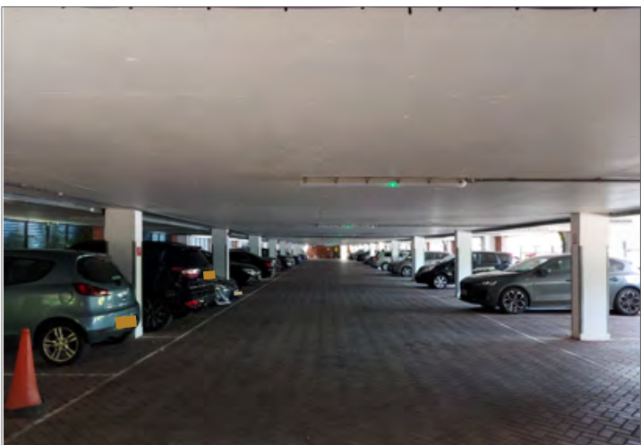
Building 9 - Parking Garage Interior view of ground floor Photograph taken 16/06/2025.
