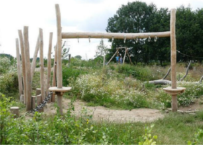
Raised, water resistant elements
