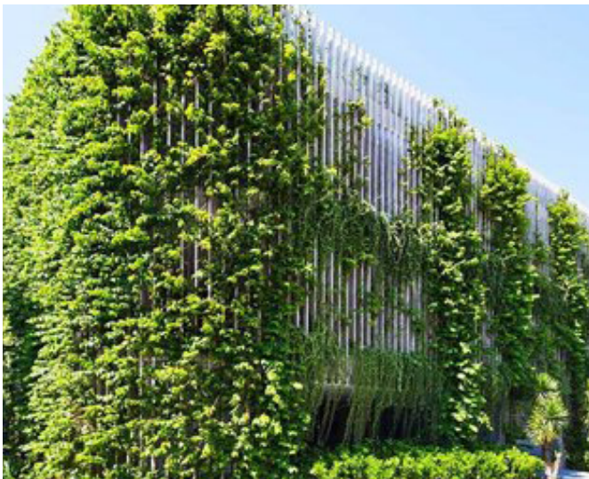
Partial vertical greening of existing car park with climbers
