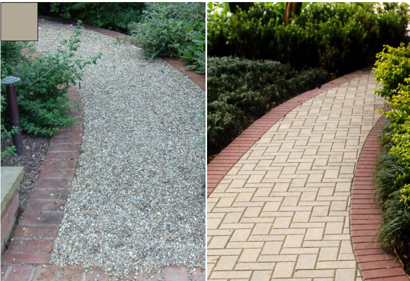
Private communal paths to be permeable block paving (south) and resin-bound gravel (north) with a brick border to provide a softer appearance and reference the brick facades
