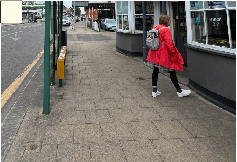
Paving following Hertsmere guidance: town and district centres use of larger (up to 900mm (w) x 600mm (l) x 63mm (d)) concrete paving with brick details in the High Street Extension area
