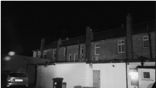
Figure 20 – B4 Position 4 – End IR view
