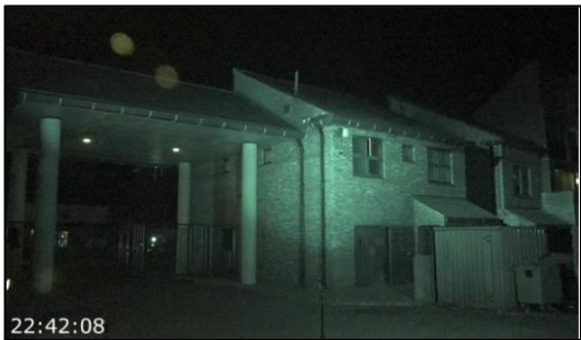
Figure 8 - B3 Position 4 – End IR view
