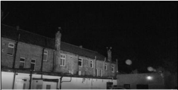
Figure 22 – B4 Position 5 – End IR view
