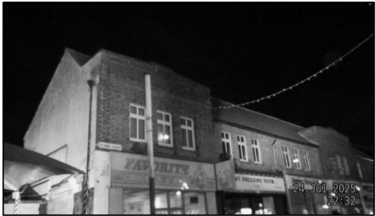
Figure 14 – B4 Position 1 – End IR view
