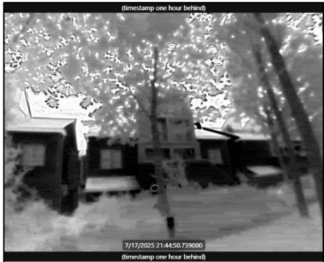
Figure 12 - B3 Position 6 – End IR view
