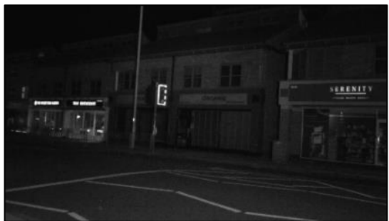
Figure 4 - B3 Position 2 - End IR view
