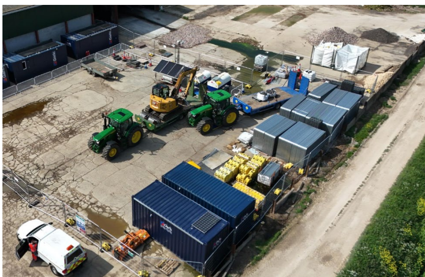
Figure 3: A temporary compound used for ground investigation works.
