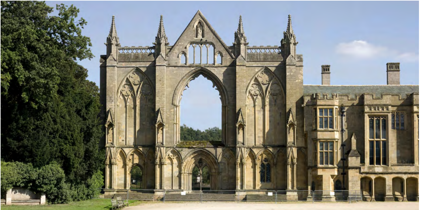
Grant funding of £103,000 was given for repairs at Newstead Abbey, the former Nottinghamshire home of Lord Byron.
