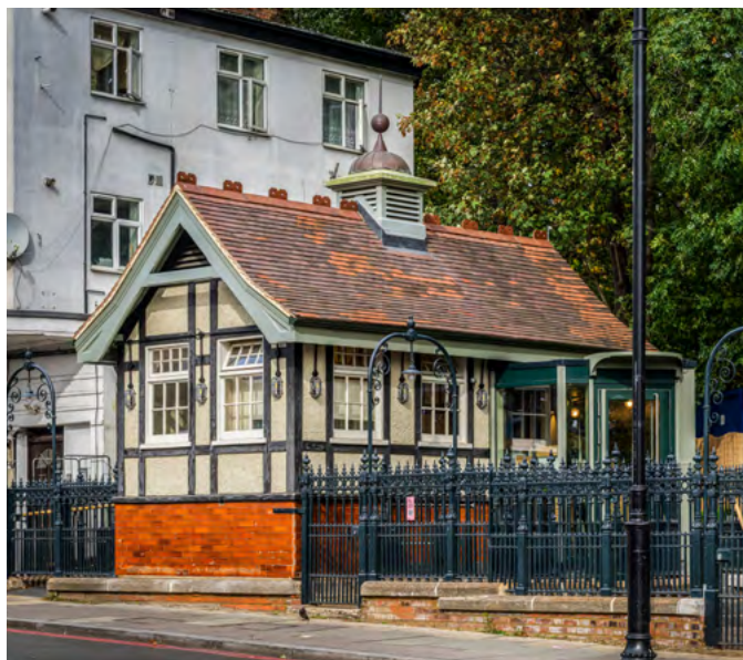
Bruce Grove Public Toilets in Tottenham, London were brought back into re-use as a café and community space.
