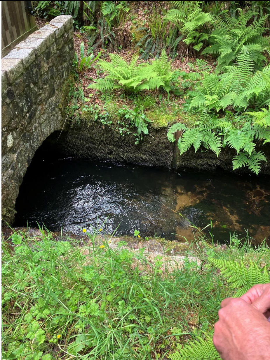
Fig 4.0 Discharge, tail race and drum screen fixing channels.
