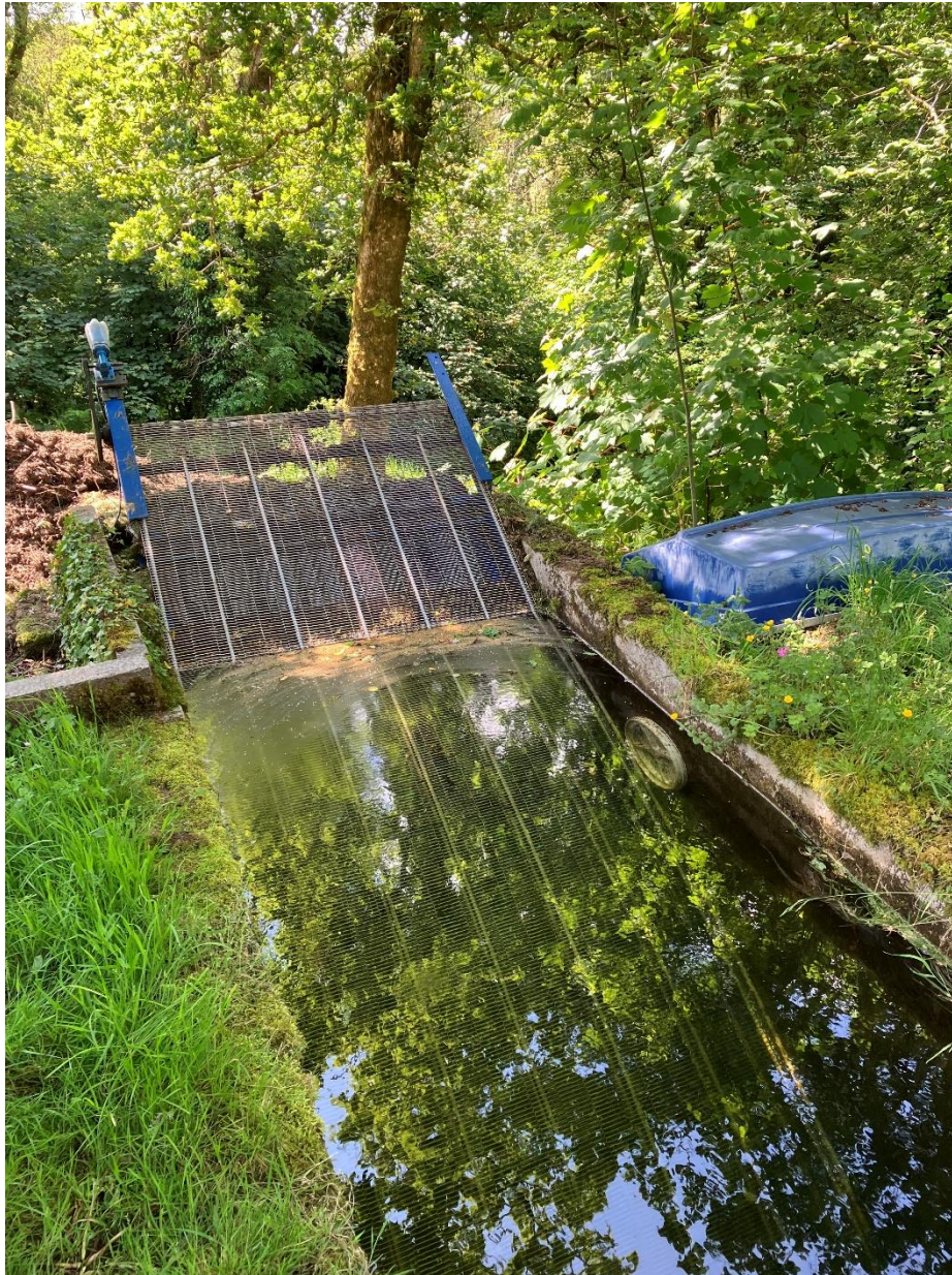
Fig 3.0 Screen and bywash channel opening (white cap).
