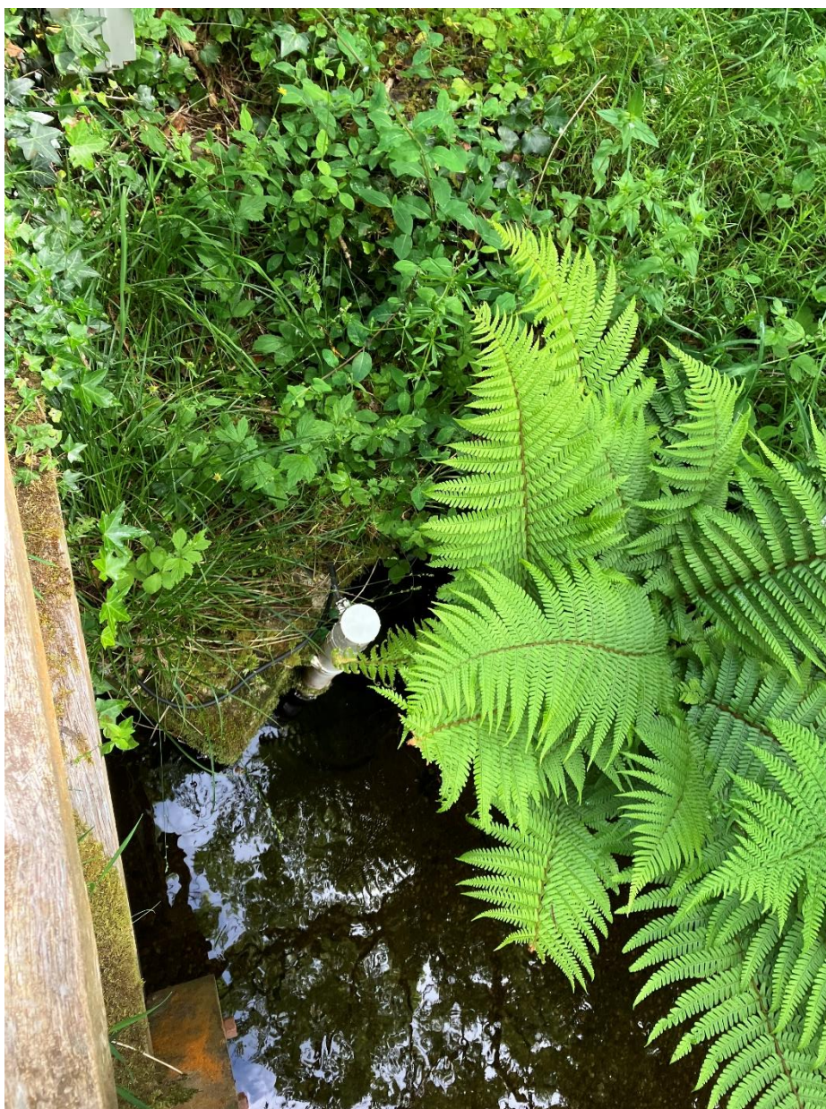
Fig 1.0 Level sensor location at intake.
