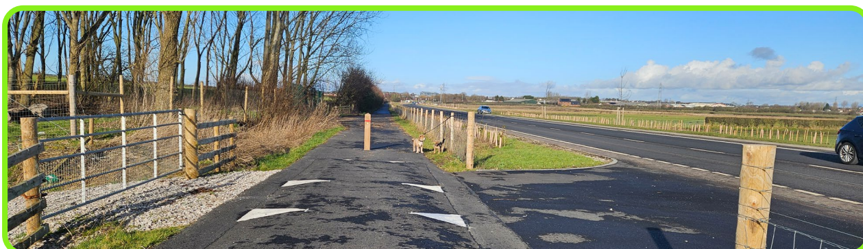
Figure 5: New shared path with speed humps and bollards.
