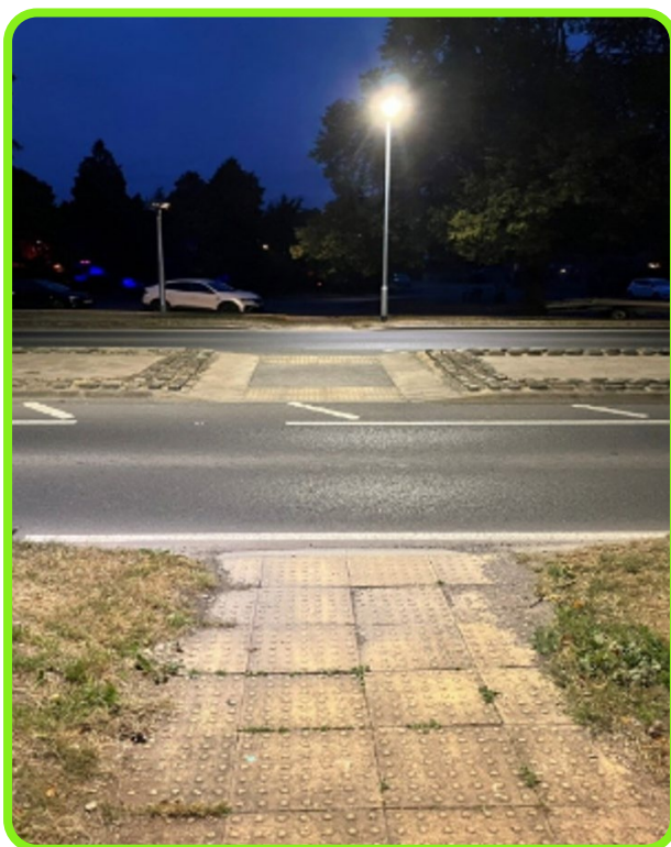
Figure 1: Example of lighting only on the crossing point, Hayton.
