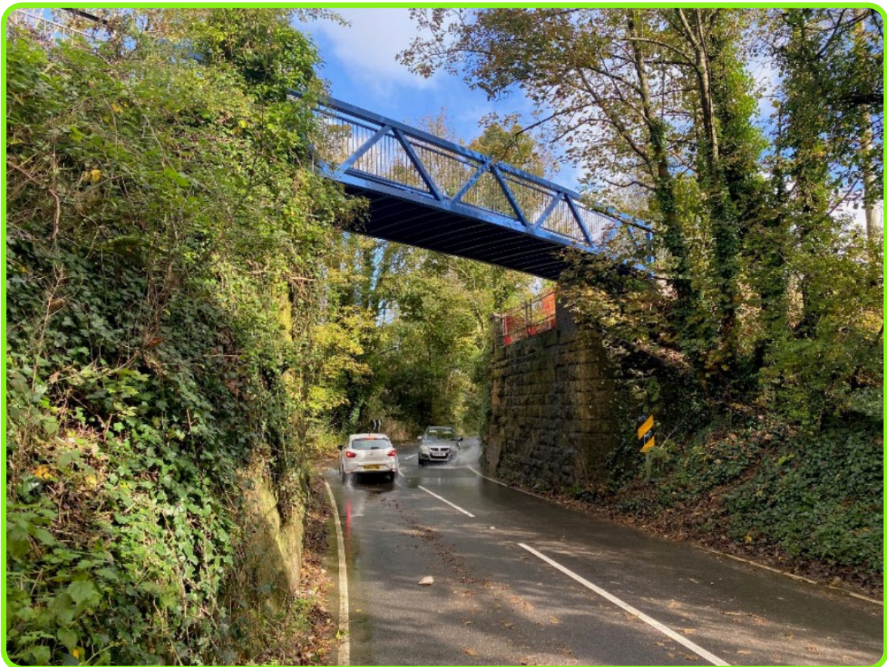
Figure 10: New bridge over the B3134 at Shepton Mallet.
