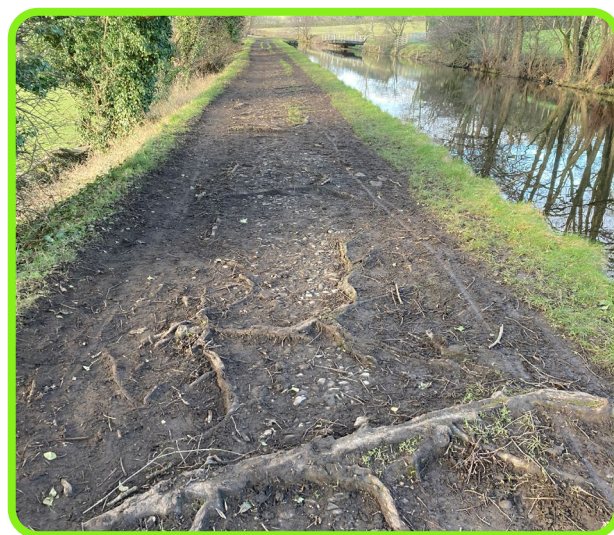
Figure 5: 'Before' example of tree roots safeguarded through surface construction method.
