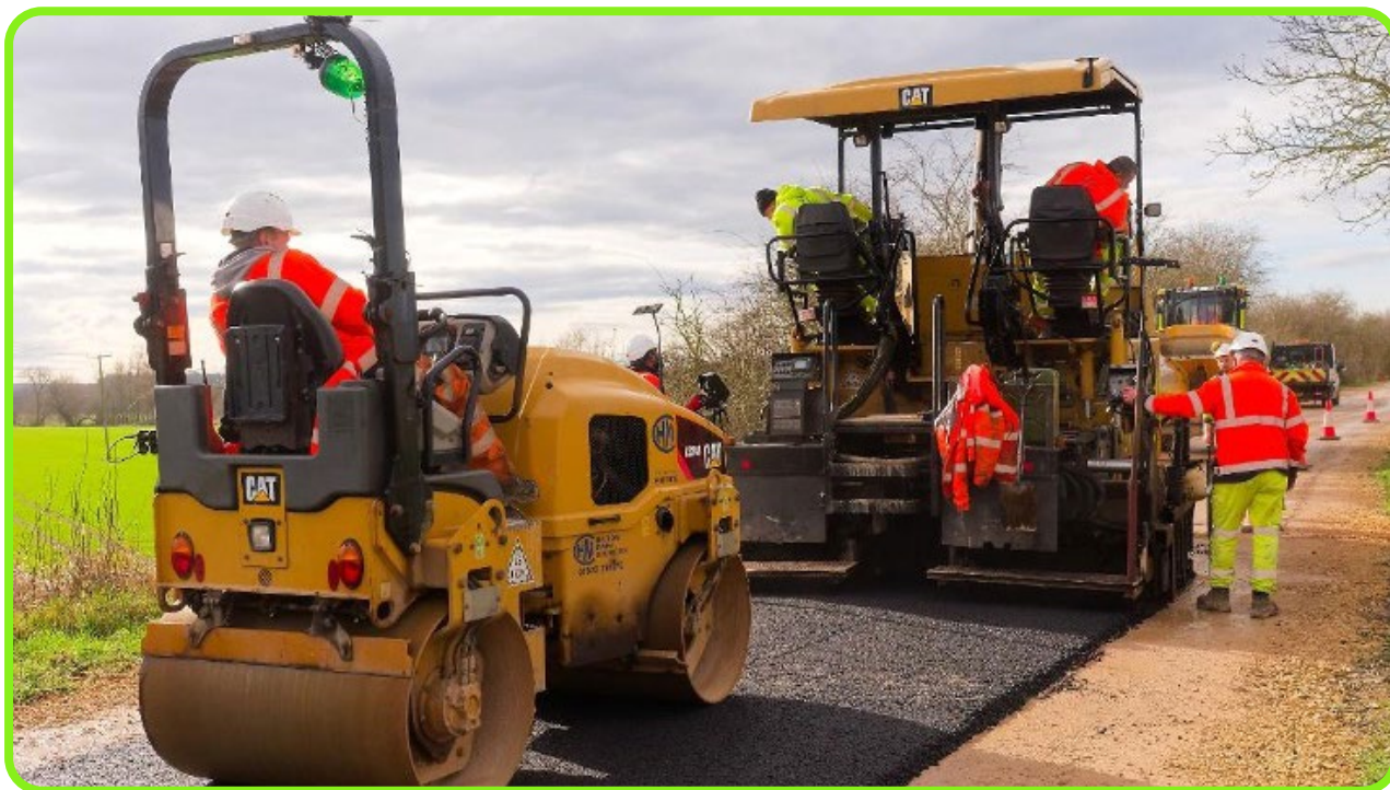
Figure 8: Installation of machine-laid asphalt on the Lias Line.
