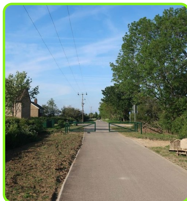
Figure 9: Completed resurfacing on Mere Way.
