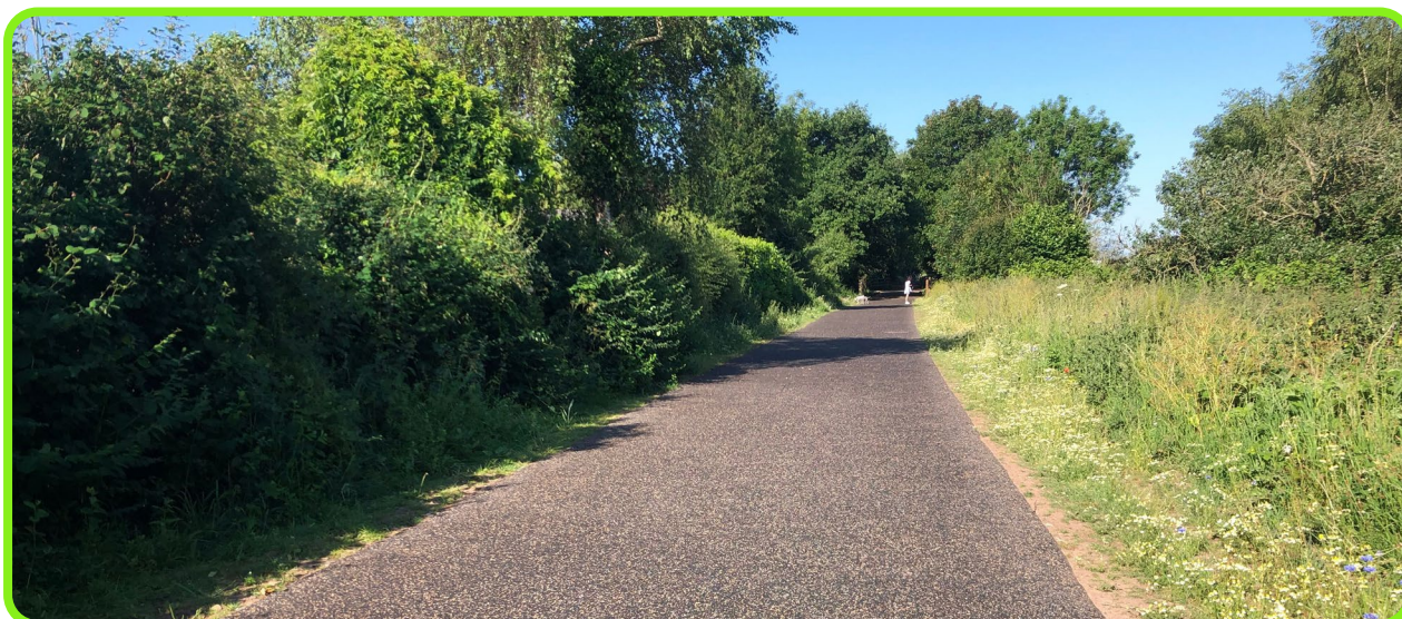
Figure 5: Newly installed flexipave surface on the Trans Pennine Trail.
