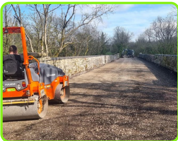
Figure 4: Hamwood viaduct, Somerset Circle.
