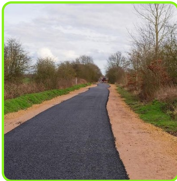
Figure 4: Newly installed asphalt on the Lias Line, with trotting strip provided either side.
