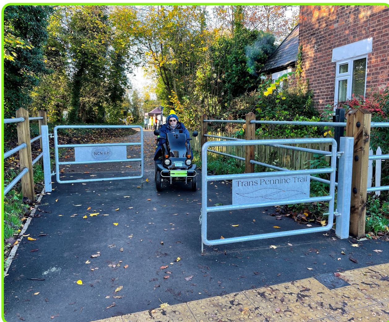
Figure 6: Access controls on the Trans Pennine Trail upgrade.
