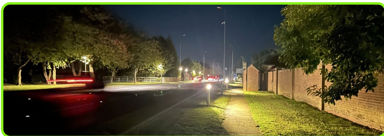
Figure 3: Current highway standard lighting visible in background, with project lighting visible lower, and illuminating the footway more than the carriageway.
