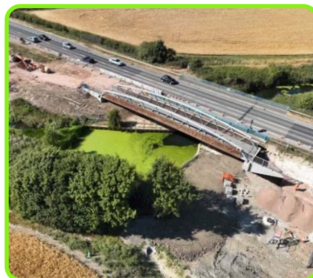
Figure 10: The new bridge was installed across the River Cuckmere in 2022 ahead of schedule.
