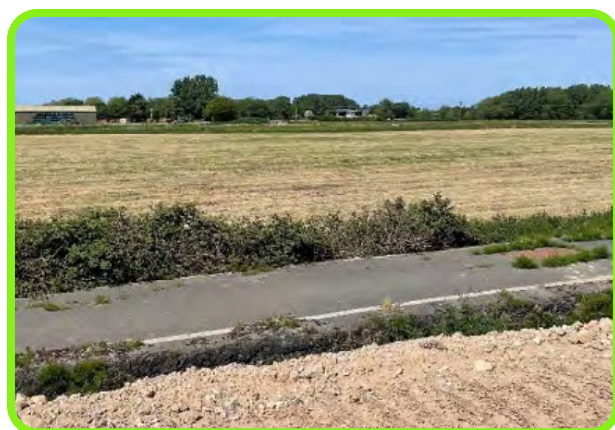
Figure 7: Wild Lane prior to resurfacing and upgrade.
