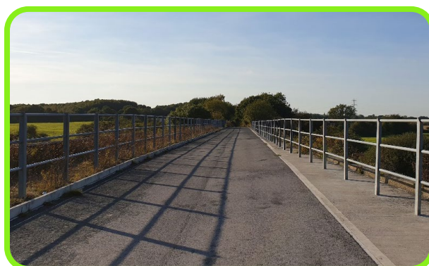
Figure 6: Refurbished bridge across the River Calder.
