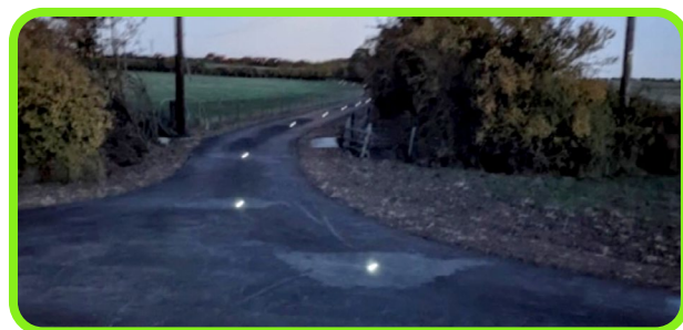
Figure 8: Solar stud lighting on St Peter's Greenway at dusk.
