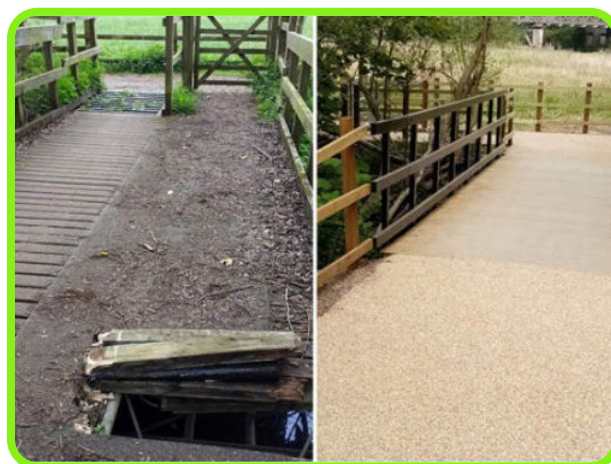
Figure 5: Before and after showing renewed bridge.
