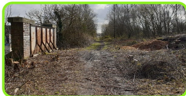
Figure 3: Former railway alignment prior to the construction of the greenway.
