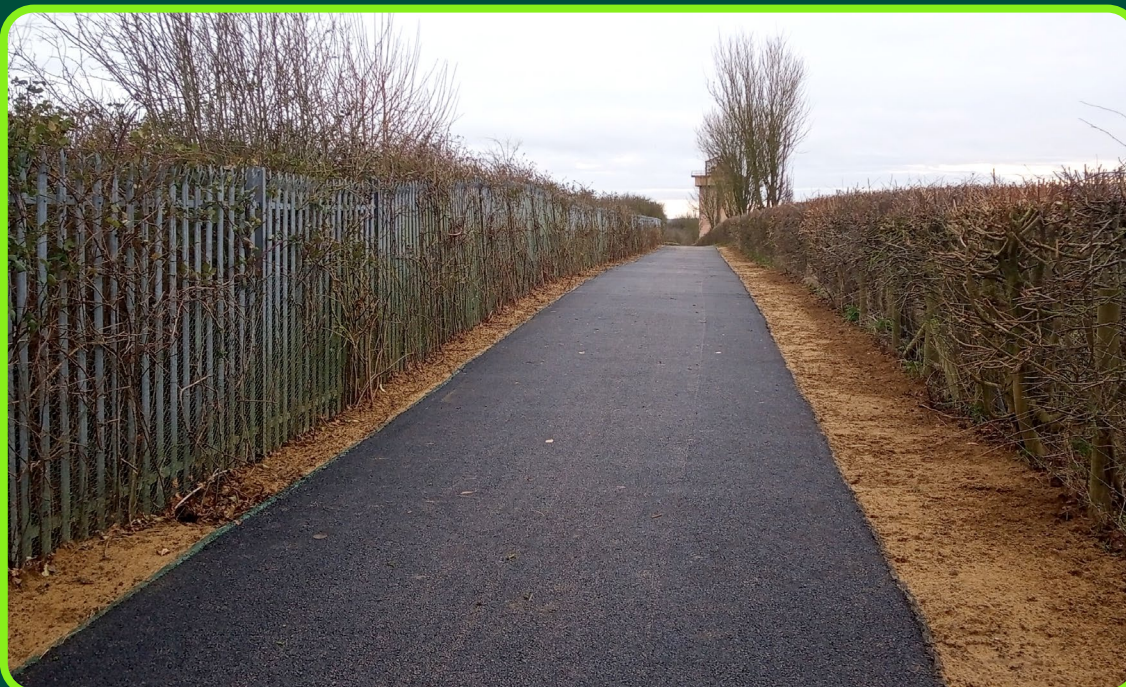
Figure 14-19: Trial of flood prevention system on the NCN.
