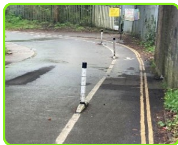
Figure 7-16: Implied footway protected by wands, Surrey.
