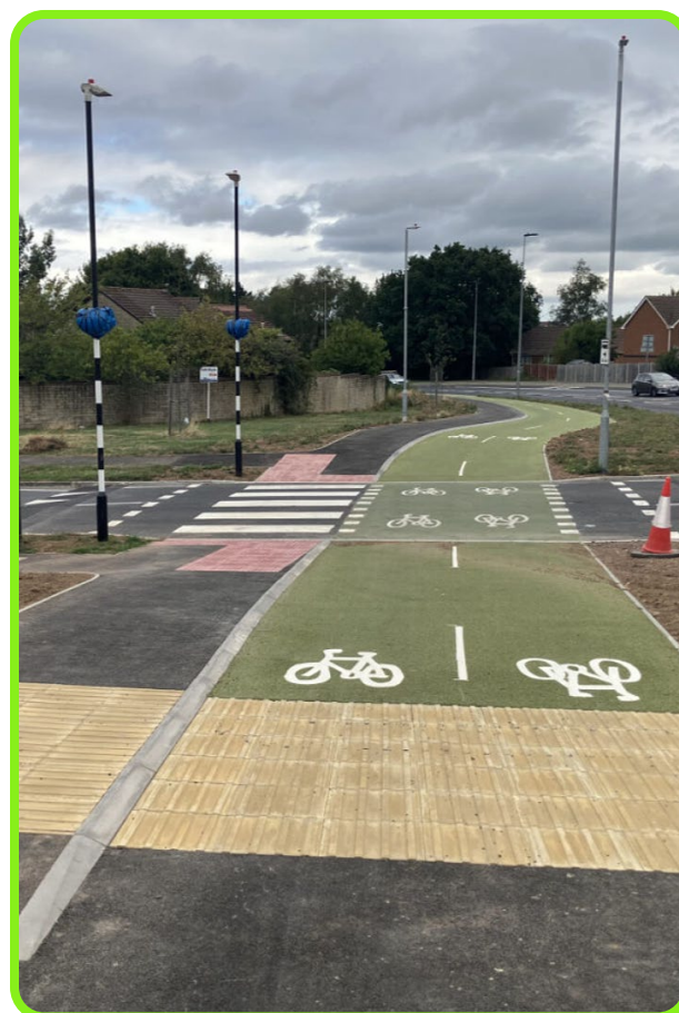
Figure 10-20: Off-carriageway route crossing minor road, South Gloucestershire.
