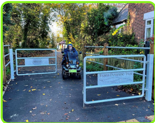
Figure 8-30: Inclusive access controls on the Trans Pennine Trail upgrade, although these would benefit from being set back further from the carriageway edge.
