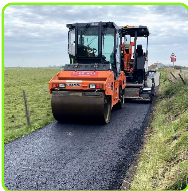
Figure 14-6: Machine-laid path construction, Rye, Sussex (Camber Road NCN 2 improvement scheme April 2022).
