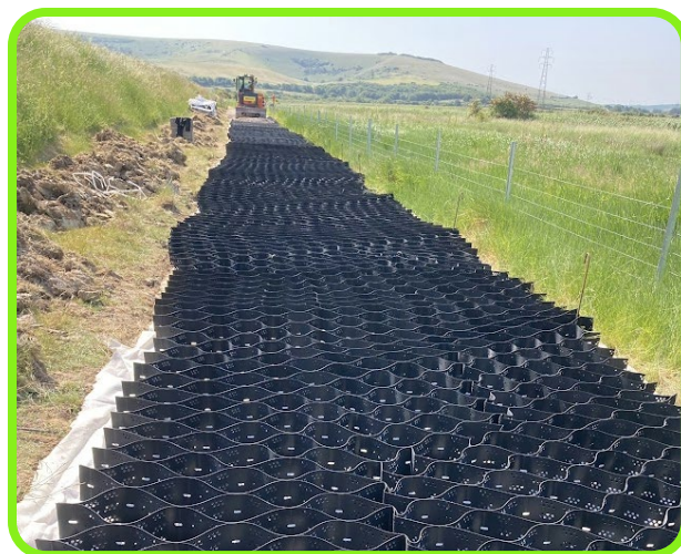
Figure 14-3: Example of geocell sub-base being constructed, Egrets Way, Sussex.
