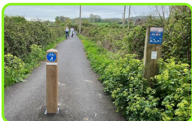
Figure 8-22: Single bollard arrangement – Flax Bourton, North Somerset.
