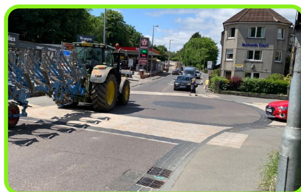
Figure 7-20: An informal roundabout in Bodmin, Cornwall.
