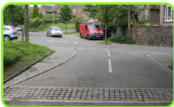
Figure 7-19: Buriton, Hampshire – tightened geometry using sympathetic materials.
