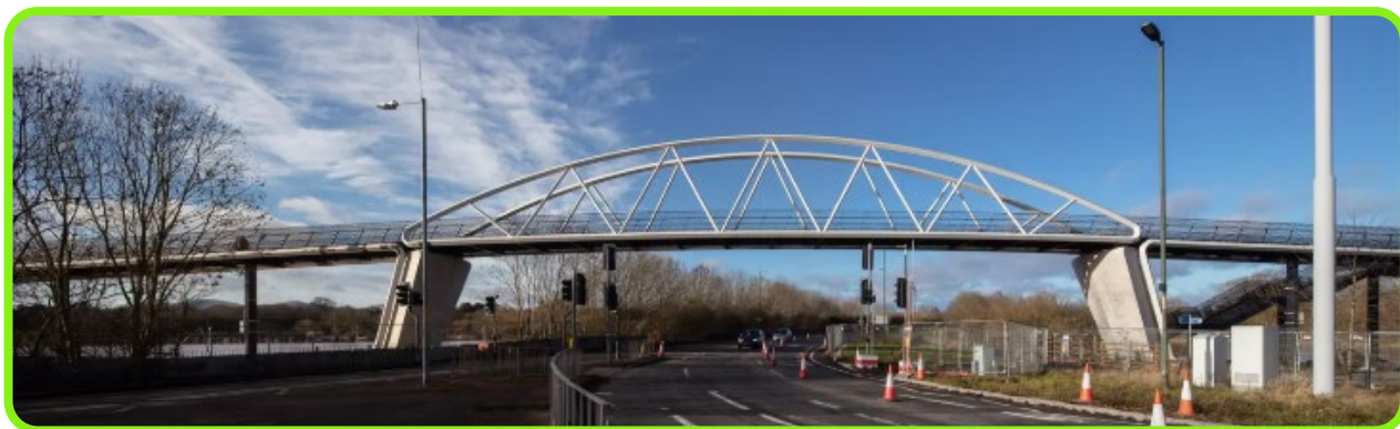
Figure 10-22: Hams Way bridge, Worcestershire.
