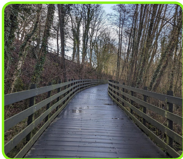
Figure 14-10: GRP boardwalk, Derbyshire.
