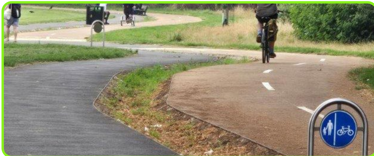
Figure 14-16: Swale drain in Bush Hill Park, Enfield, London.
