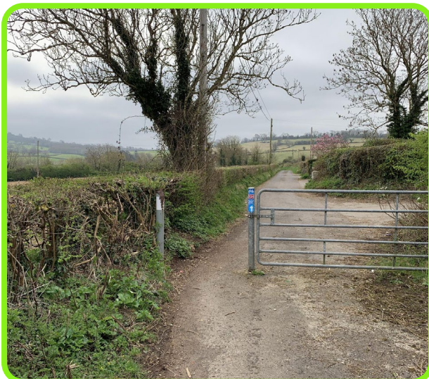
Figure 8-25: Gate and bollard arrangement – North Somerset.
