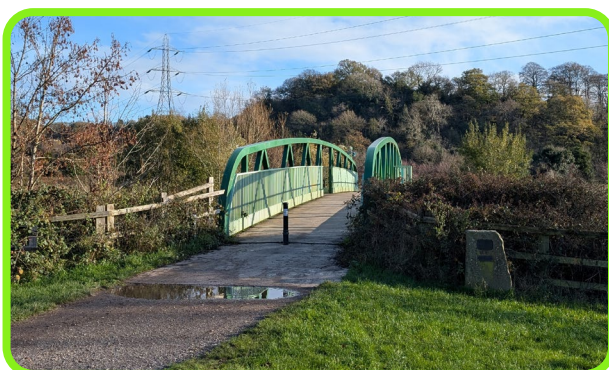
Figure 10-14: Chadkirk Bridge on NCN 55, Romiley.
