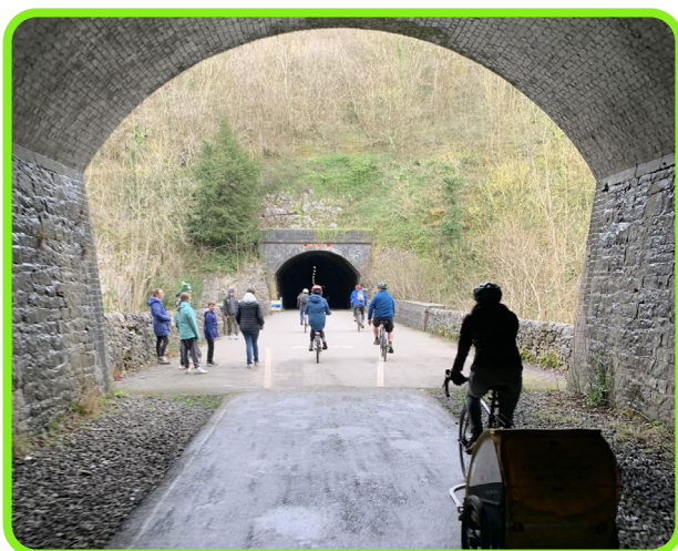
Figure 8-8: Monsal Trail along the former Midland Railway line in the Peak District National Park.
