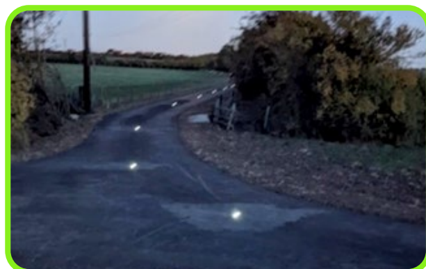
Figure 14-21: Solar stud lighting on the motor-traffic-free St Peter's Greenway, Buckinghamshire.
