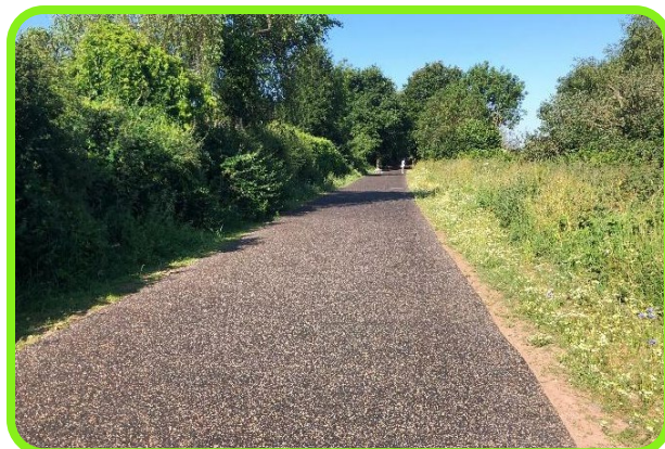
Figure 14-9: Rubber crumb permeable surface example – Trans Pennine Trail, Warrington.
