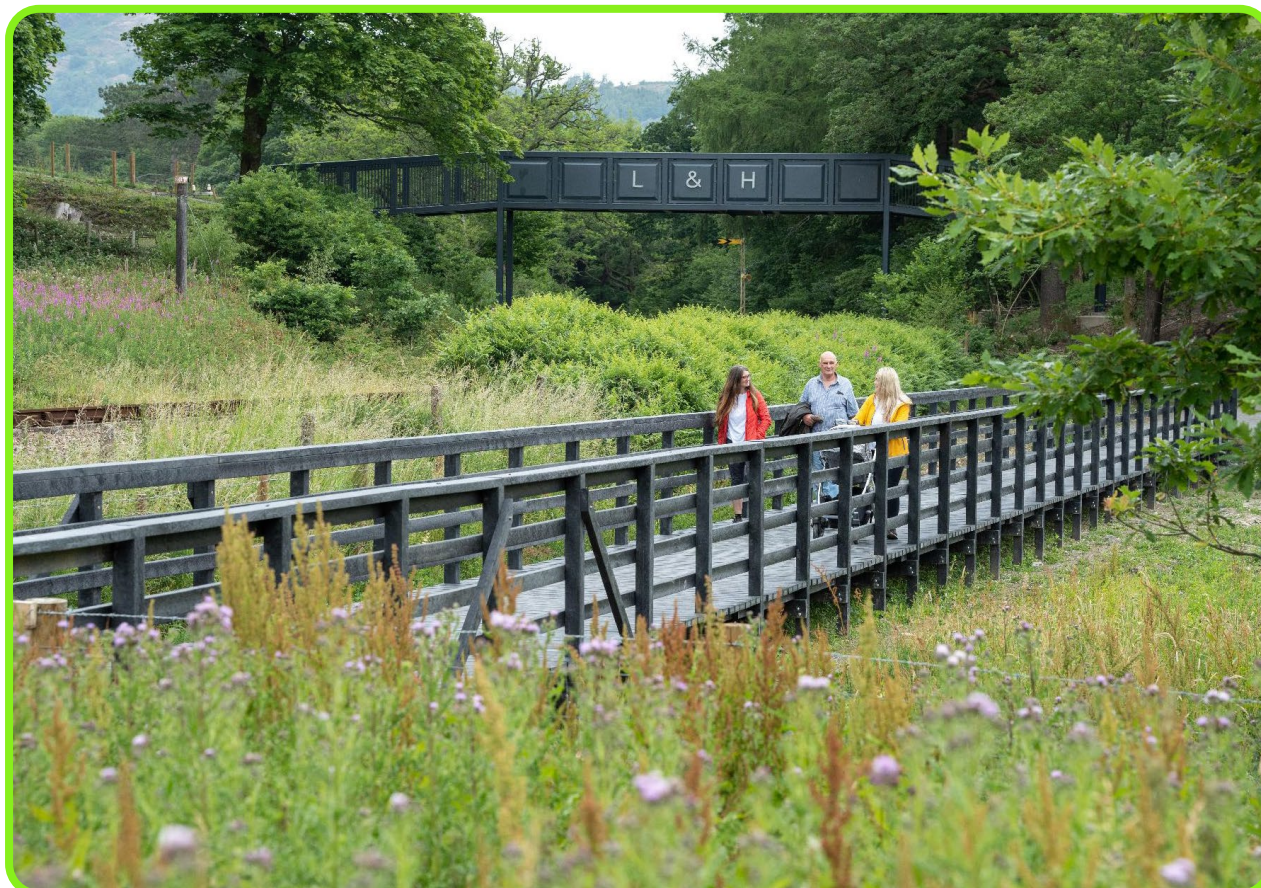
Figure 14-20: Boardwalk installed on West Windermere Way.
