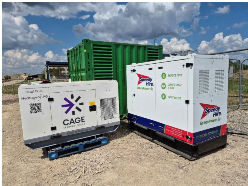
Figure 25. HGE system and Speedy battery on the HS2 Aston Le Walls site
