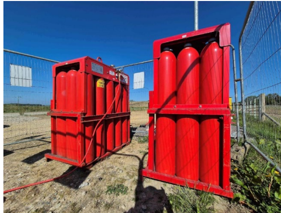
Figure 26. Hydrogen storage
