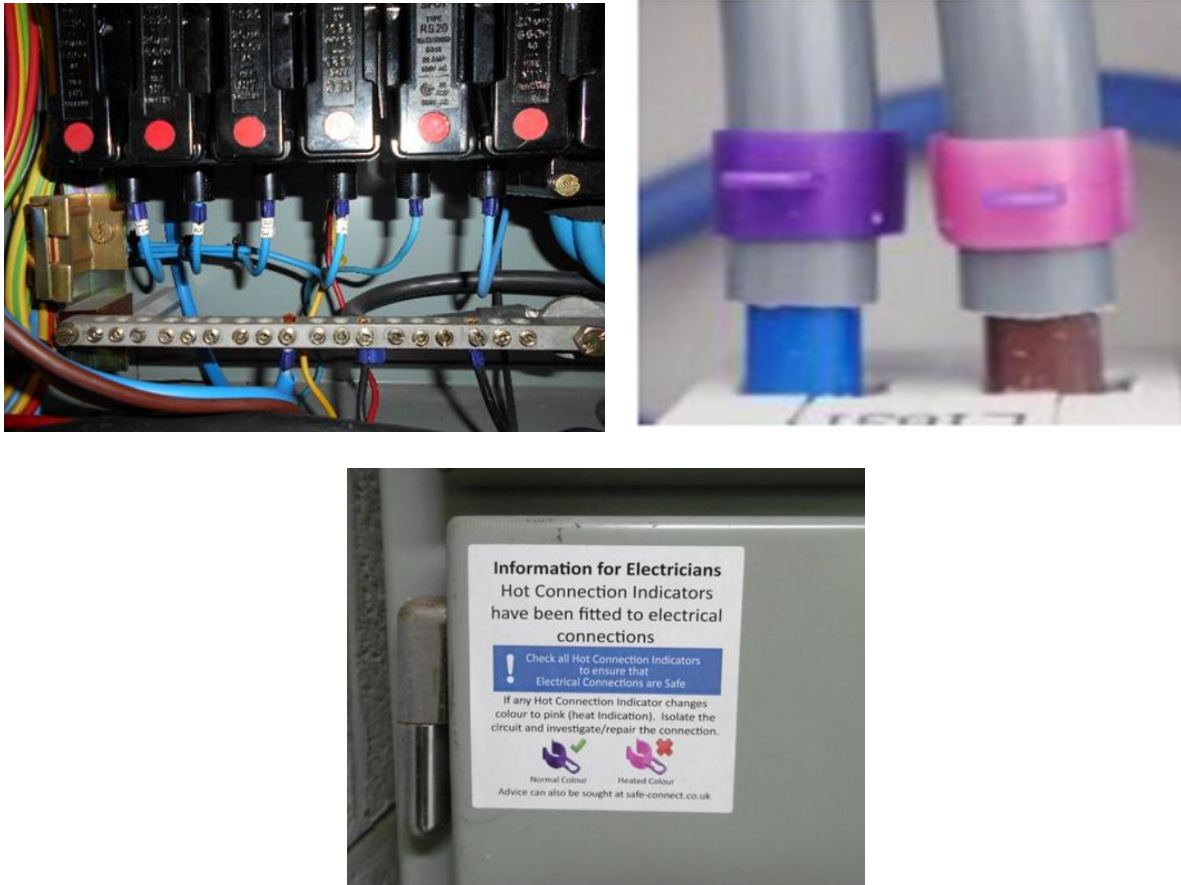
Figure 3.1: Cable hot connection indicators
