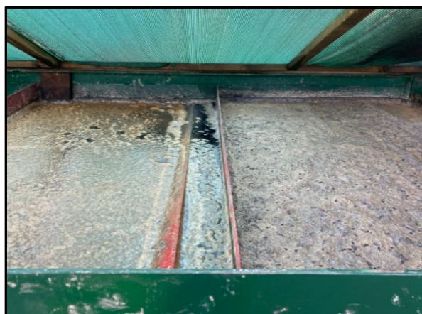
Plate 2. Oily sheen and emulsified product frequently observed in OWS (09.05.2022)
