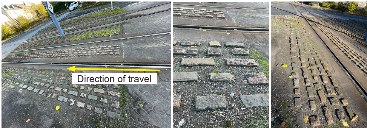
Figure 13: Cobbled surface past the footpath crossing on the outbound line at Staniforth Road footpath crossing.
