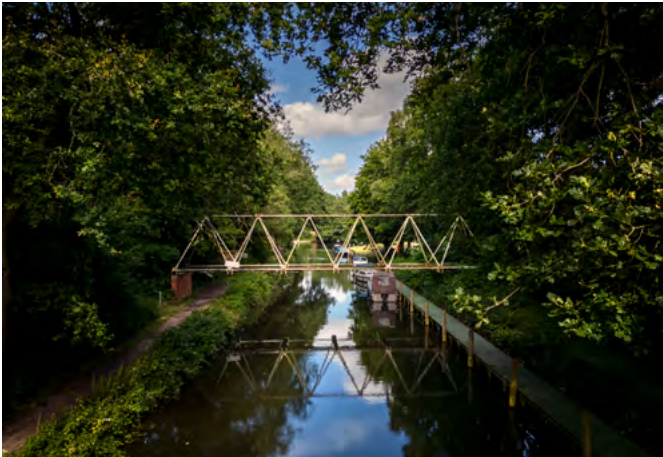
The Inglis Portable Military Bridge over the Basingstoke Canal, Aldershot, Hampshire. The component-based design allows a team of 12 soldiers to erect the structure in around 15 minutes.
