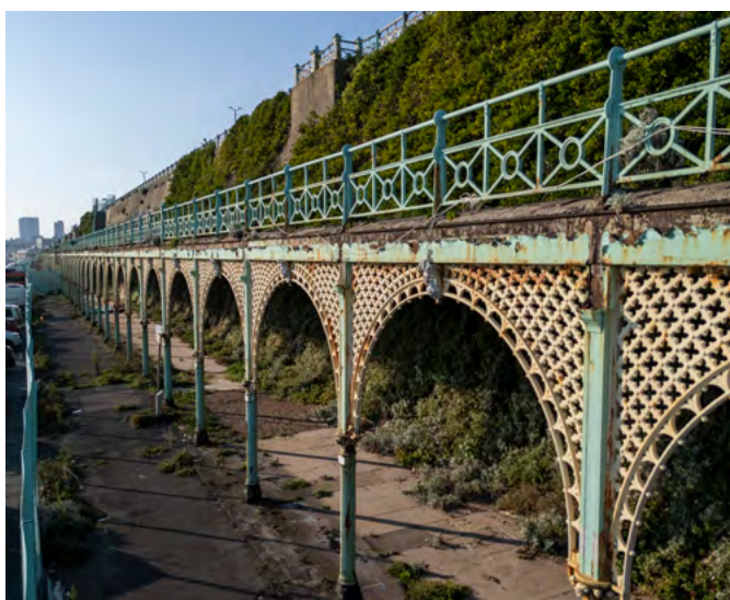
Some of the 865 metre long, cast-iron covered terrace and walkway, which forms Madeira Terrace in Brighton, East Sussex. Image shows the Terrace ahead of restoration work.
