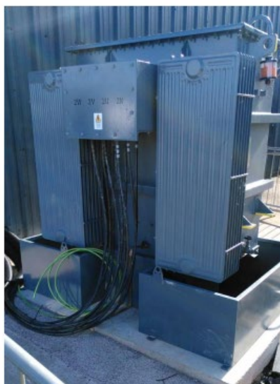
Figure 15: 11kV to 690V transformer and cabling
