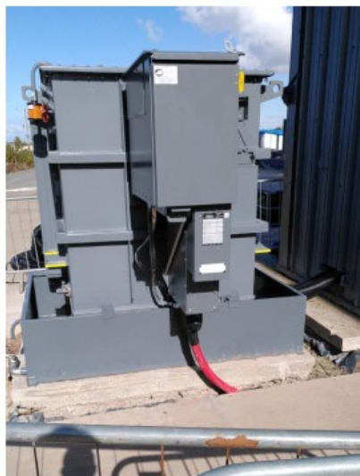
Figure 15: 11kV to 690V transformer and cabling
