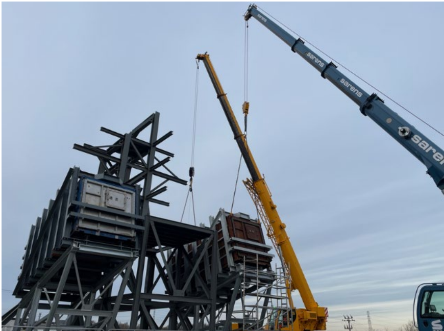
Figure 12: Silo delivery & installation
