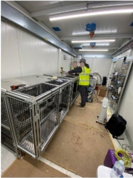
Figure 51: Installation of DU Bed frames in the MCL
