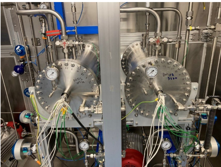
Figure 42: Beds being installed into MCL
