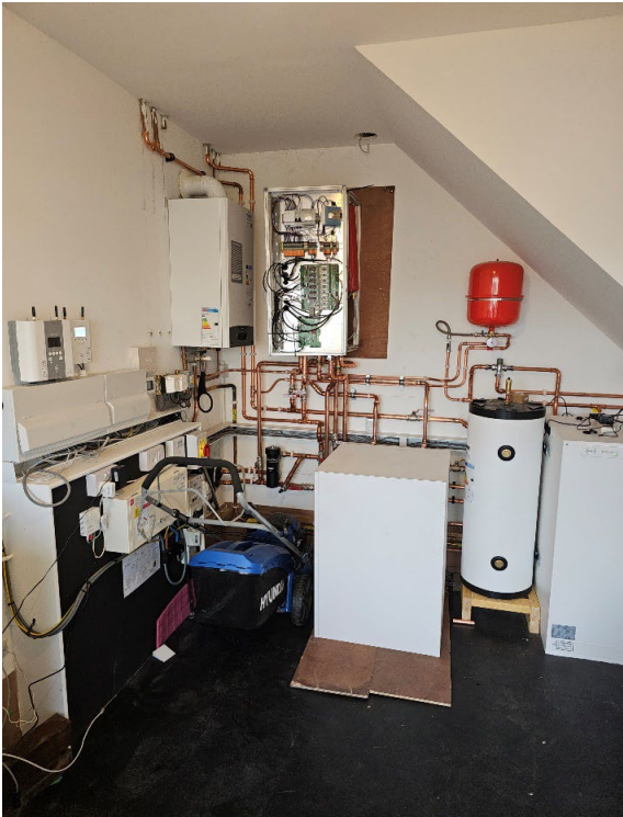
Figure 7. The EXTEND system installation in another property showing the myenegi systems and the pipework below the hydromodule.
