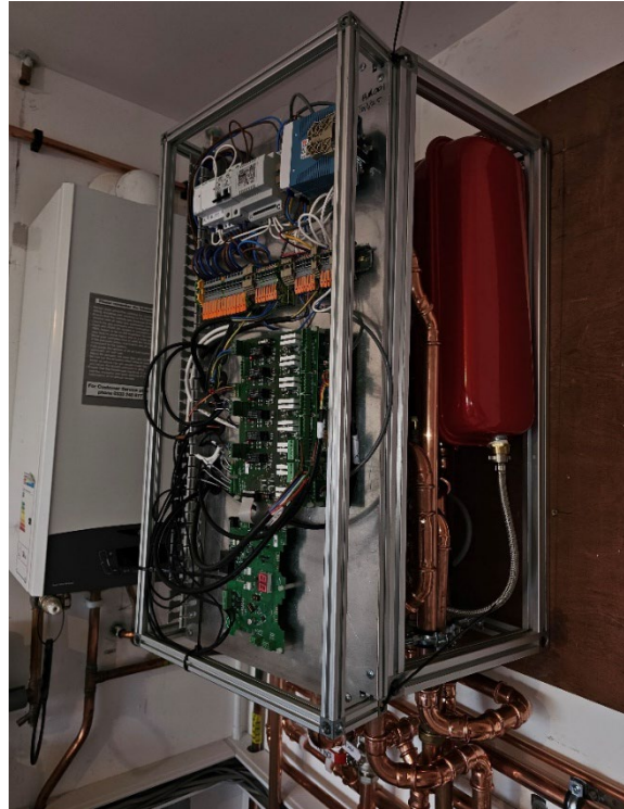
Figure 7. The EXTEND system installation in another property showing the myenegi systems and the pipework below the hydromodule.
