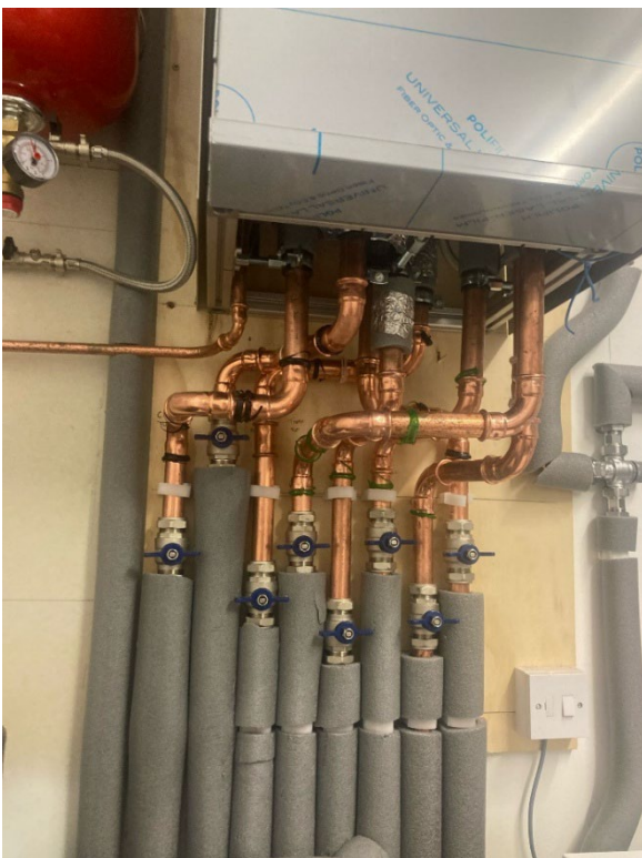
Figure 7. The EXTEND system installation in another property showing the myenegi systems and the pipework below the hydromodule.
