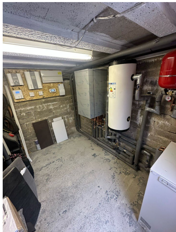
Figure 7. The EXTEND system installation in another property showing the myenegi systems and the pipework below the hydromodule.
