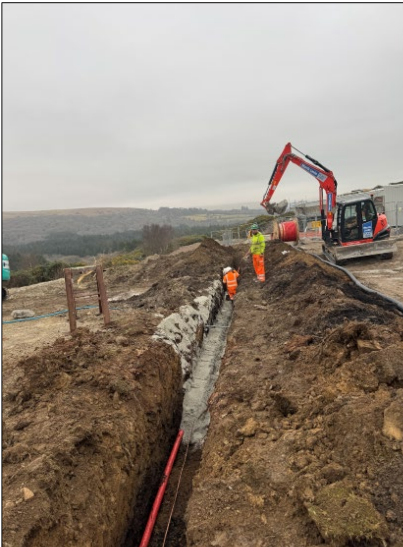
Figure 22 Running the HV cable
