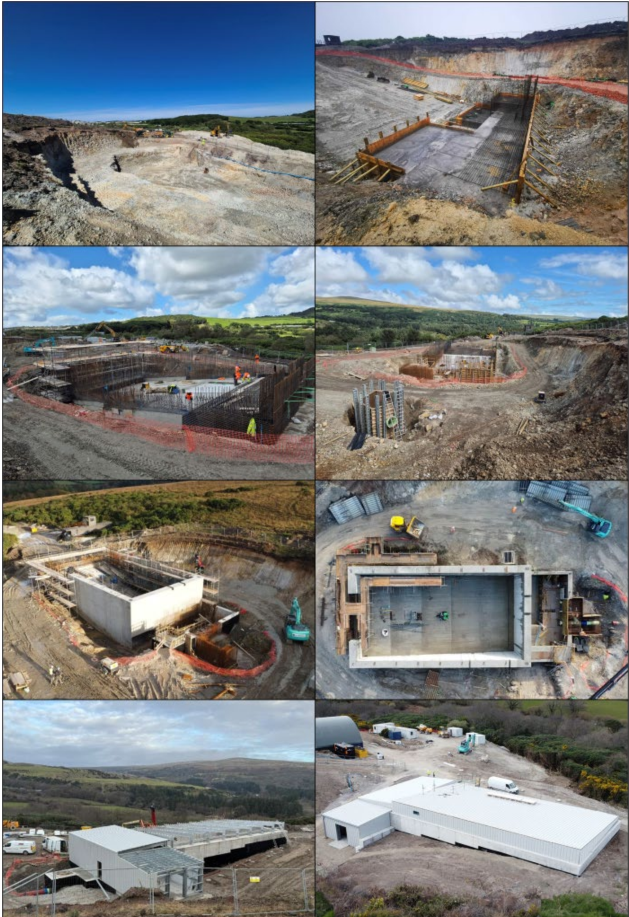
Figure 18 Lower reservoir and powerhouse construction
