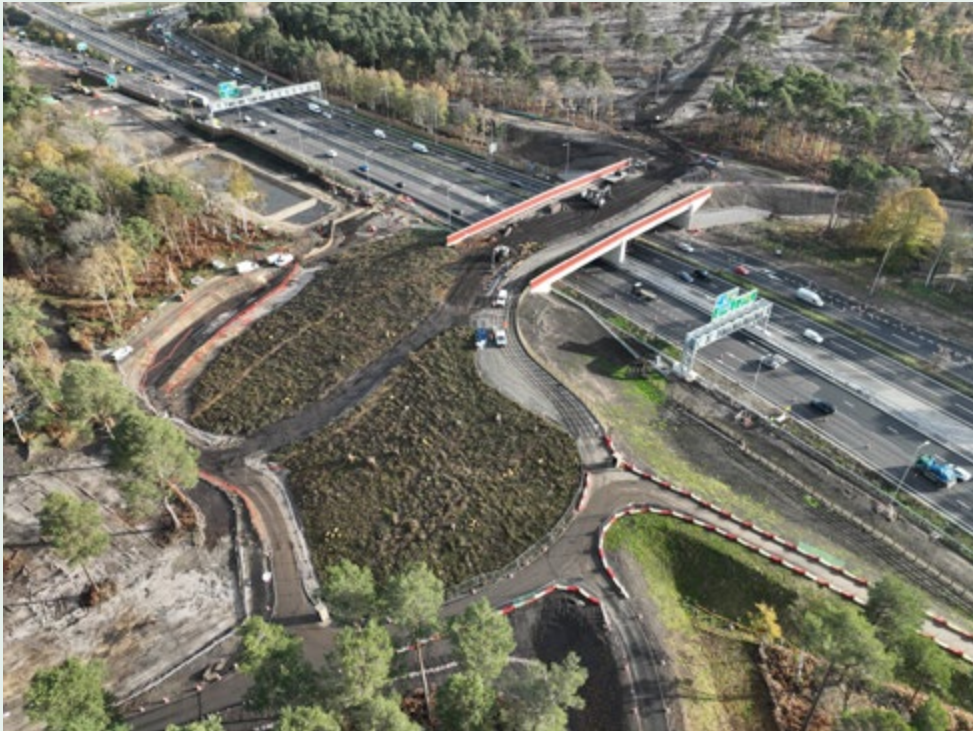
Figure 7: Cockrow Green Bridge (Source: National Highways)
