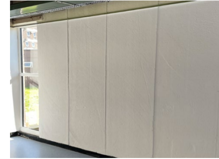
Figure 5: Example of RAAC to an internal wall face
