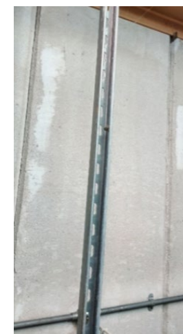
Figure 9: V-shaped grooves at 600mm spacing
