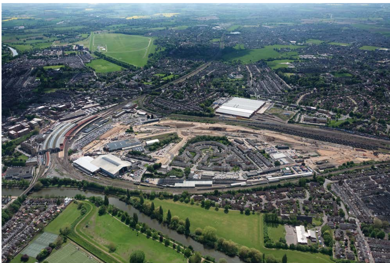
An aerial view of the carriage works site at York Central
