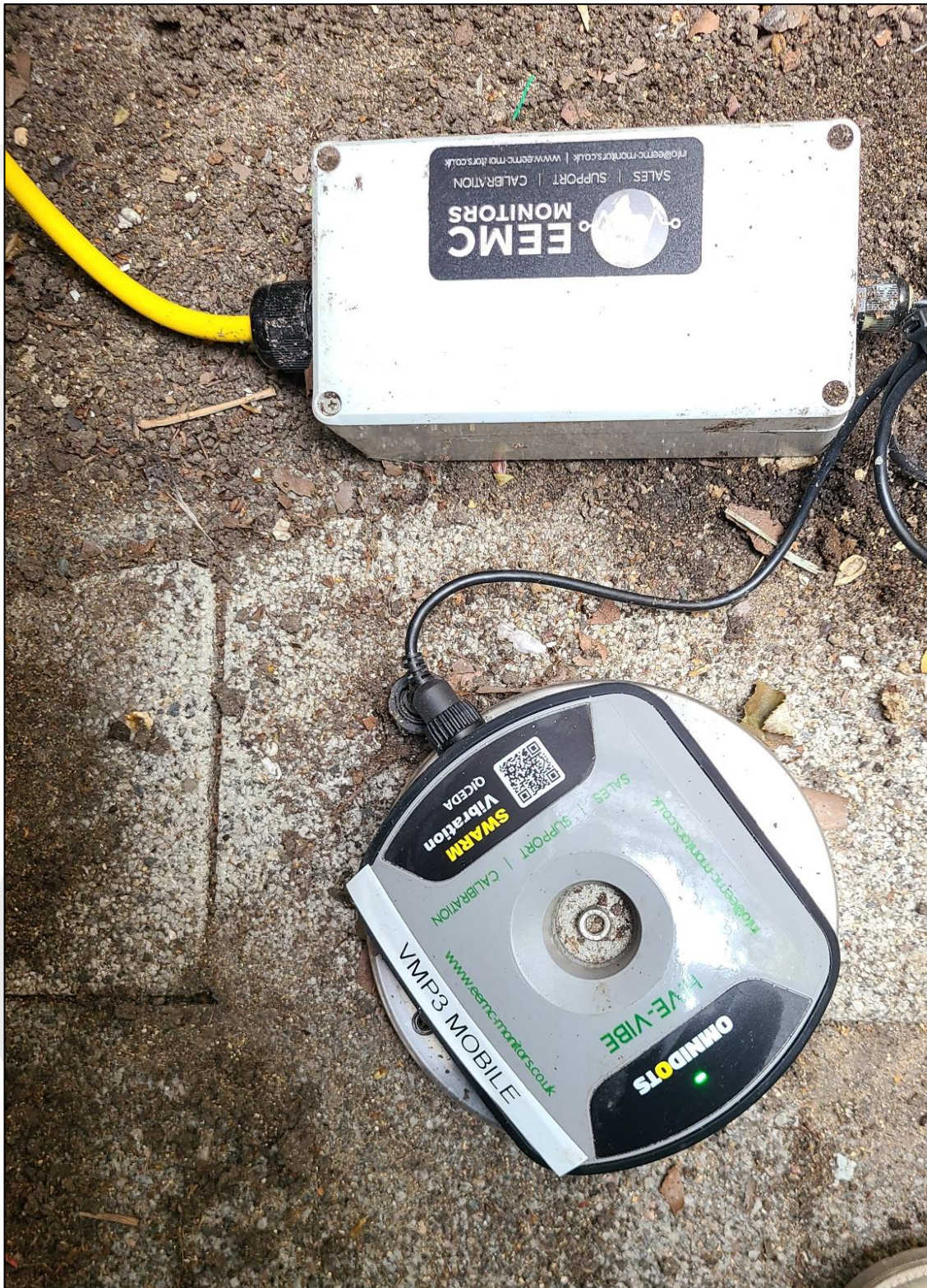
Image 4 – VMP3 Monitoring Location
