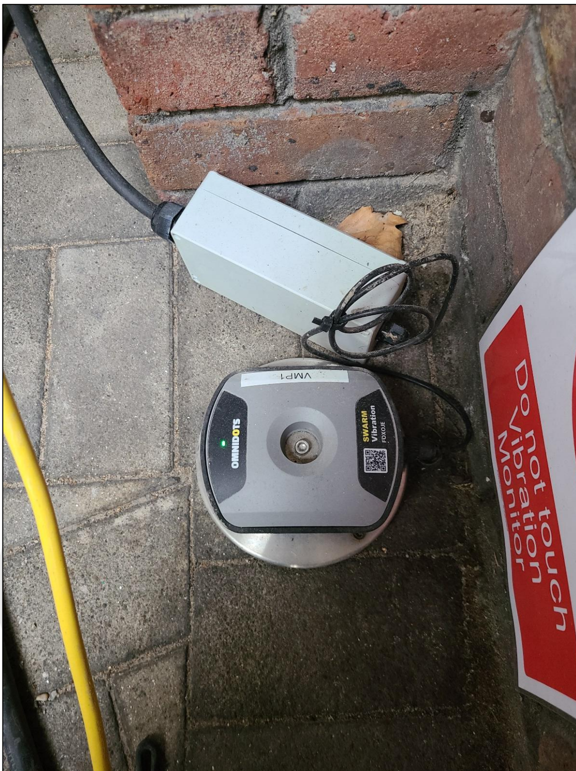
Image 2 – VMP1 Monitoring Location
