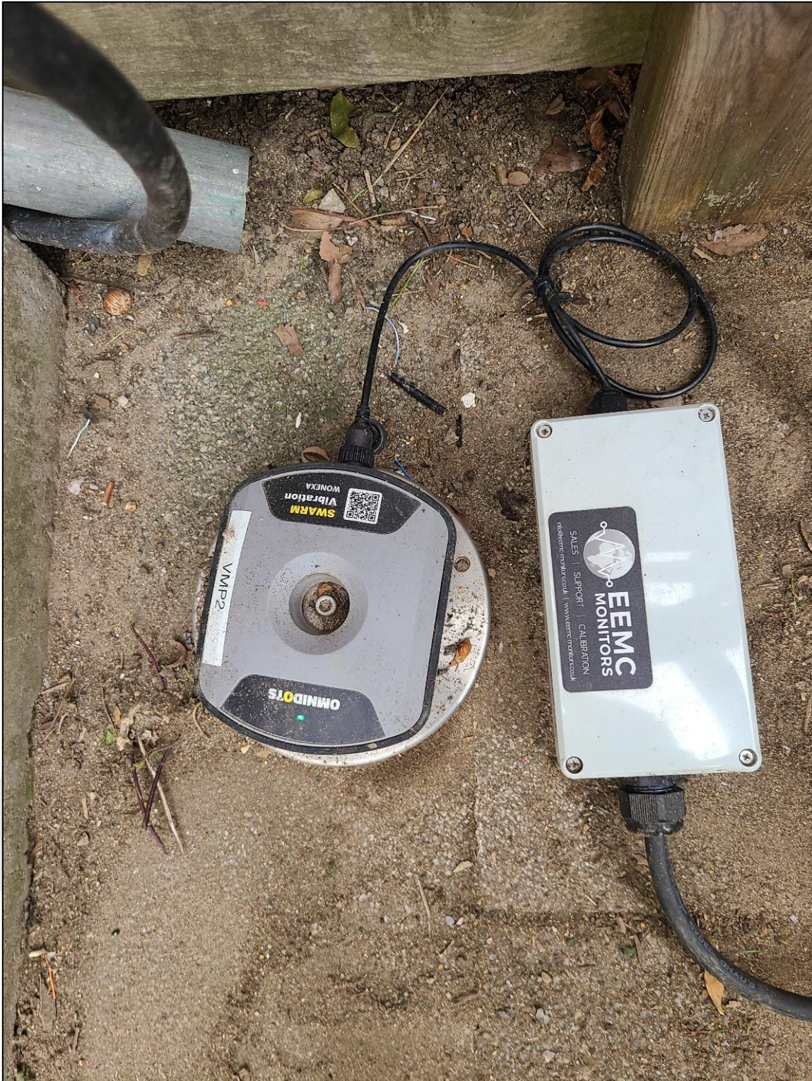
Image 3 –VMP2 Monitoring Location
