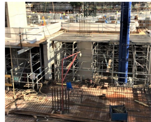
Figure 5: Example of a concrete-framed school building
