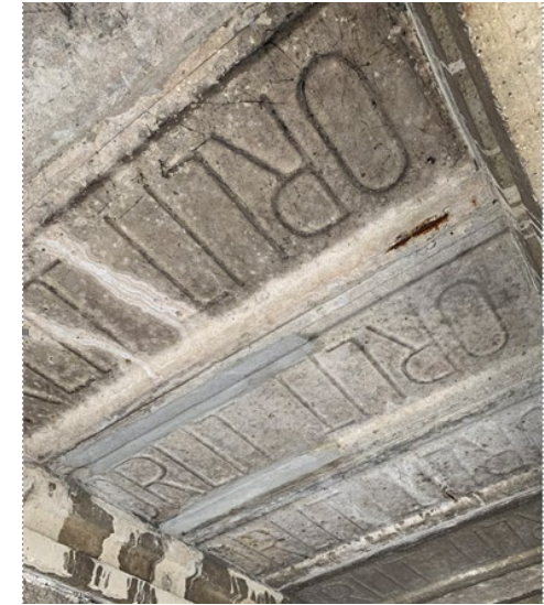
Figure 16: Example of an Orlit soffit
