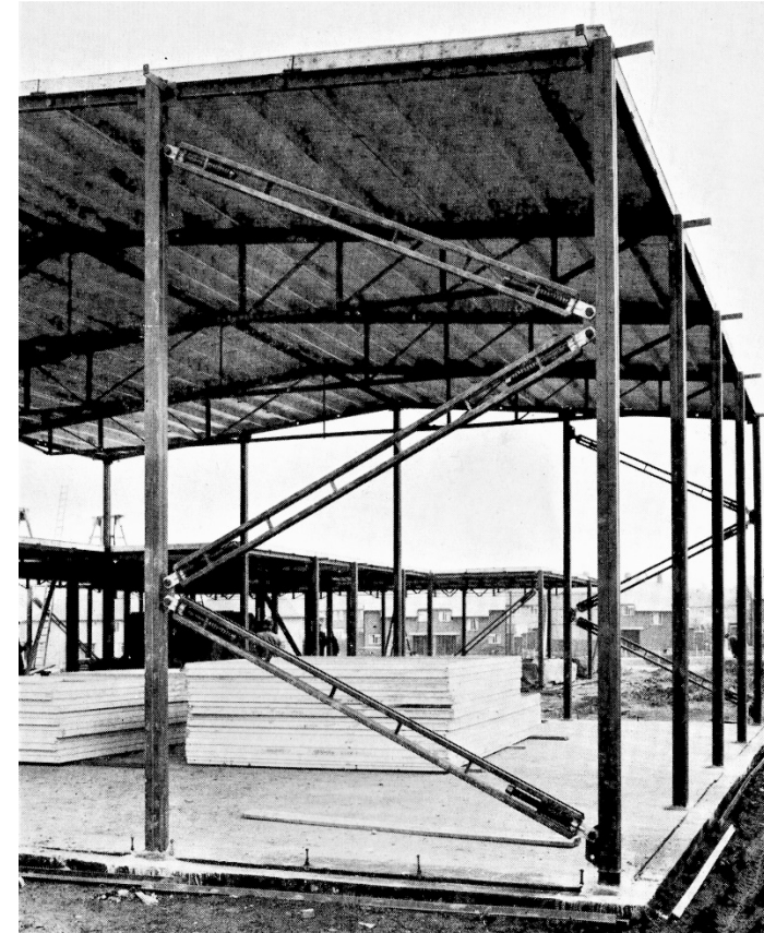
Figure 3: Example of a post-war CLASP system school building with a modular frame
