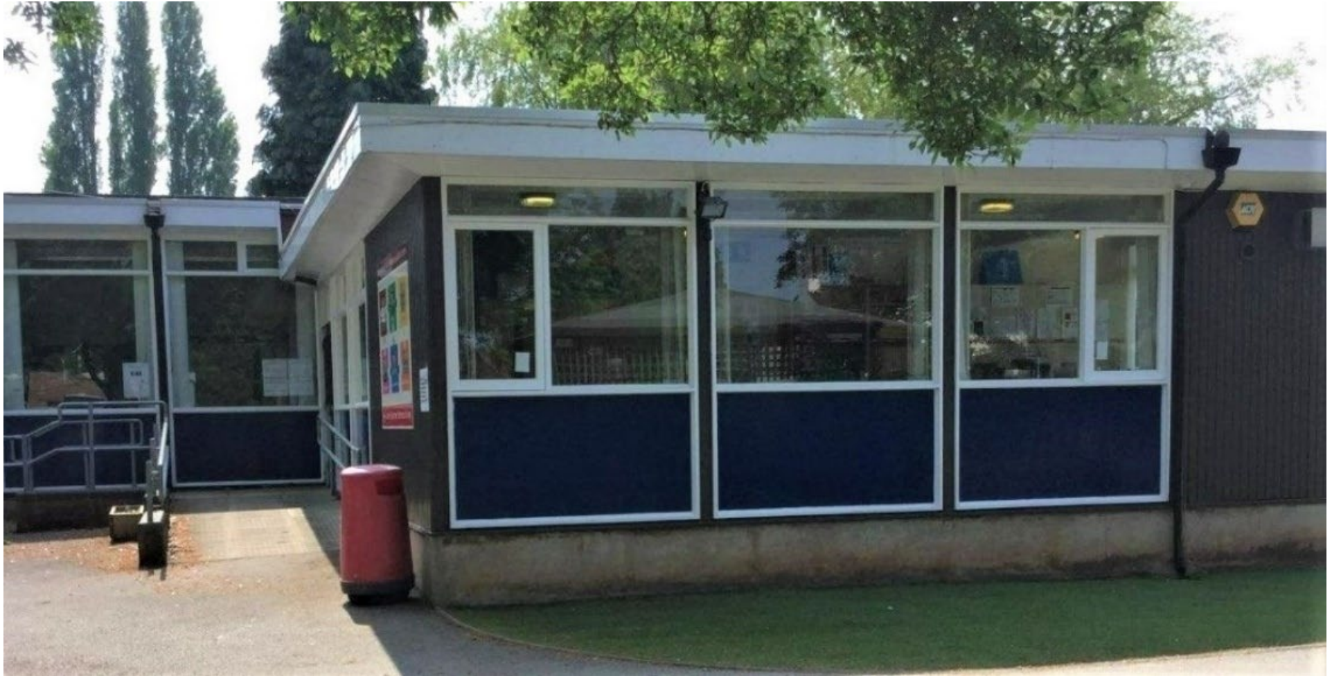
Figure 8: Example of a Derwent system school building with panelised external cladding
