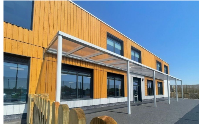
Figure 6: Example of a completed modular school building using modern methods of construction
