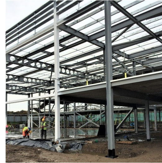
Figure 4: Example of a steel-framed school building
