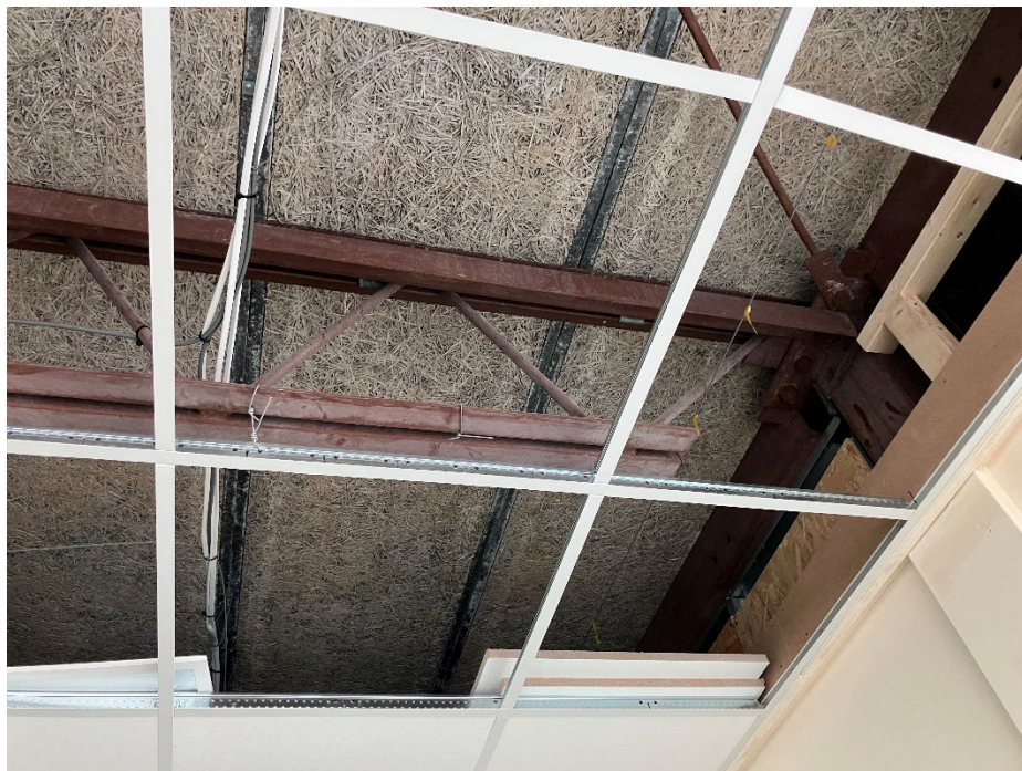
Figure 40: Woodwool roof slab supported by steel trusses
