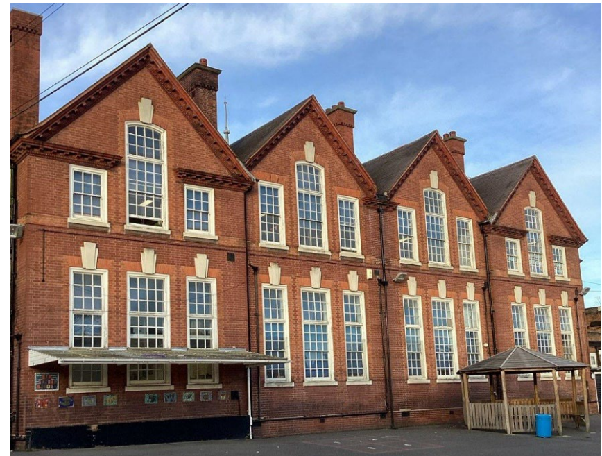
Figure 1: Example of a traditional pre-war school building constructed from masonry with a pitched roof and chimney features
