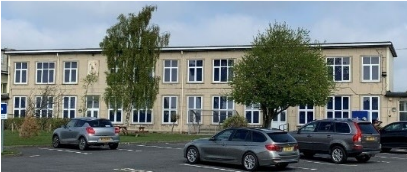
Figure 15: Example of an Orlit system school building with a precast concrete frame and panel construction
