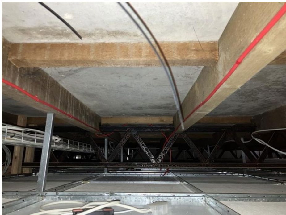
Figure 41: Example of a TonkinDek slab roof system constructed from composite board materials
