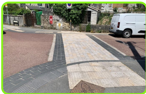
Figure 7-21: Courtesy crossing, Bodmin.
