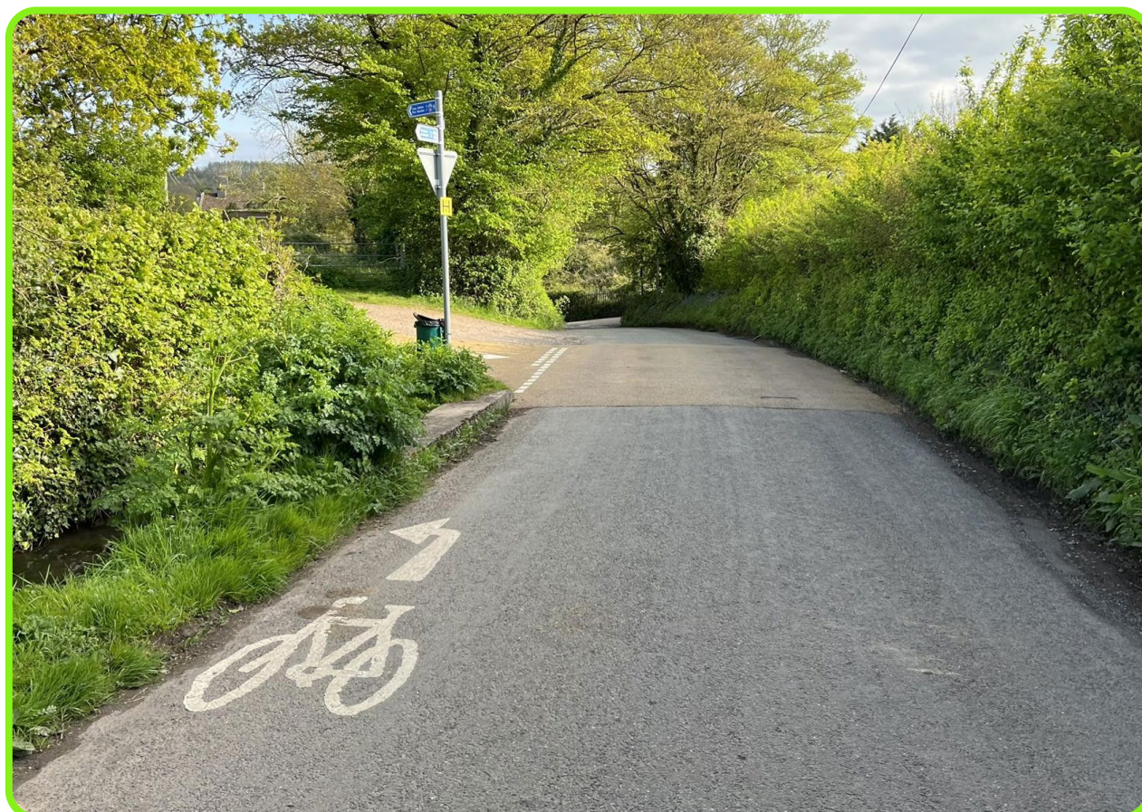
Figure 12-18: Surface dressing, carriageway markings and signing combine at the transition between traffic-free and mixed traffic sections, providing advanced warning to route users and drivers.
