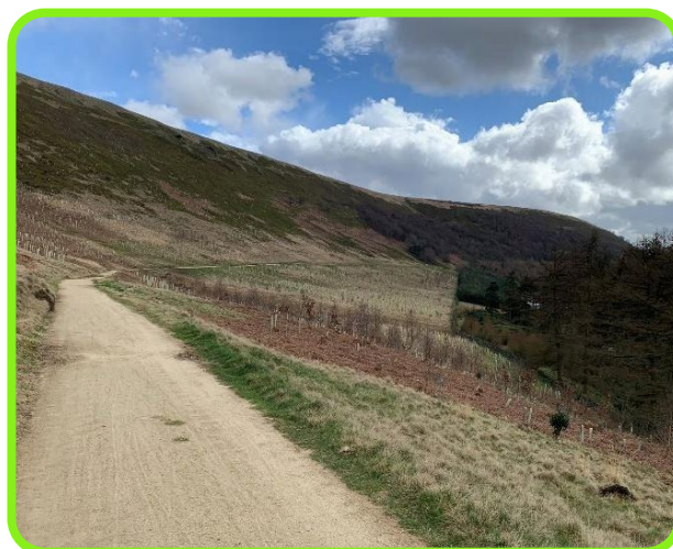
Figure 14-4: Hoggin path along a bridleway in the Peak District National Park.
