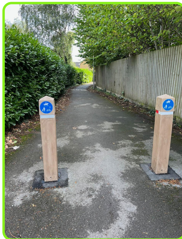
Figure 8-23: Double bollard arrangement – Nailsea, North Somerset.
