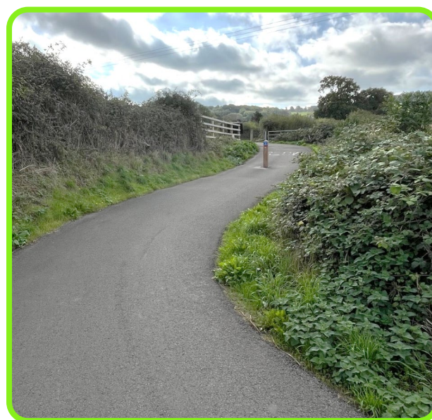
Figure 10-5: Path turns through two 90-degree bends on approach to crossing with path marking to highlight the need to slow and give way.
