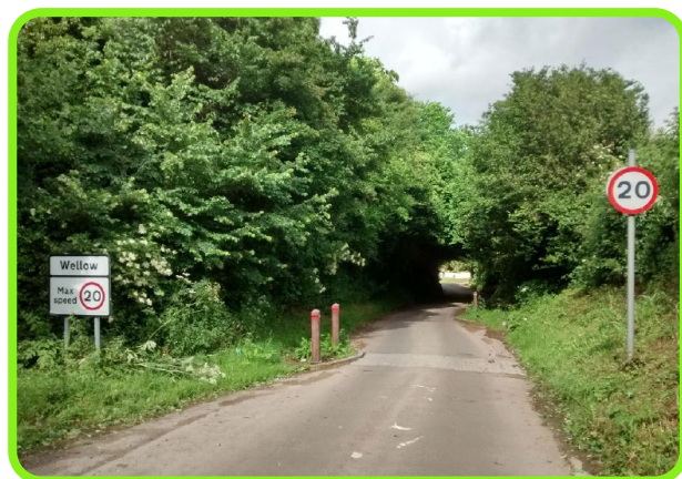
Figure 7-7: Informal build-outs with bollards and local change in surfacing.
