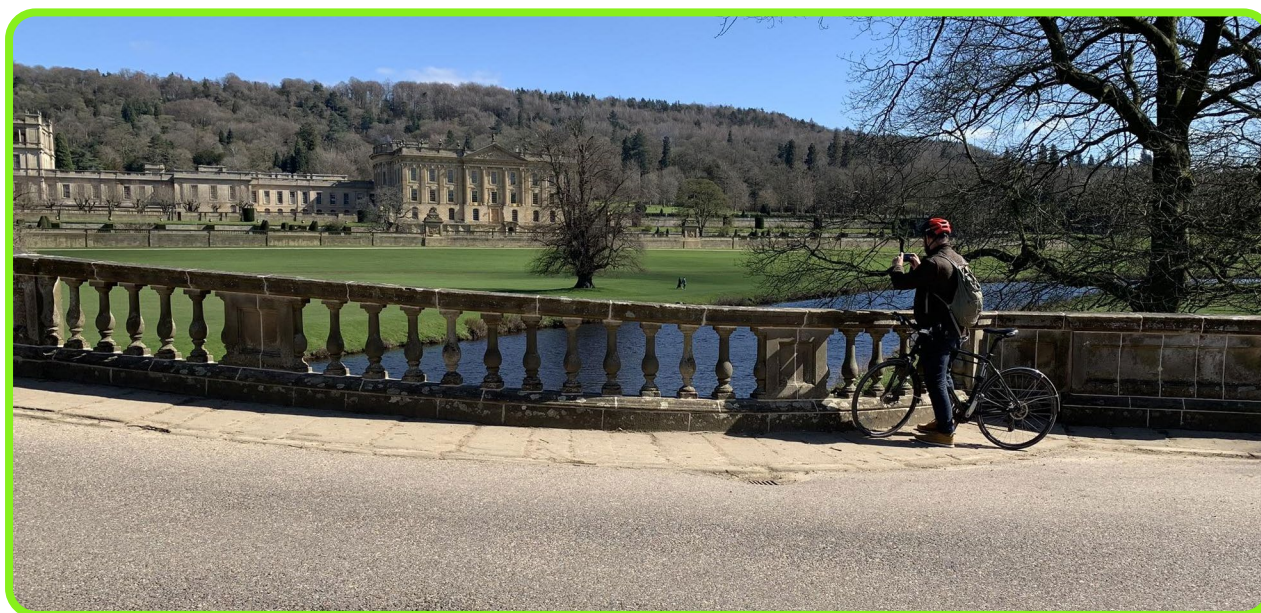
Figure 8-20: Chatsworth House, Derbyshire.
