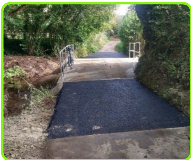
Figure 7-3: Improvements to Rydon Lane, Exeter Green Lanes case study.
