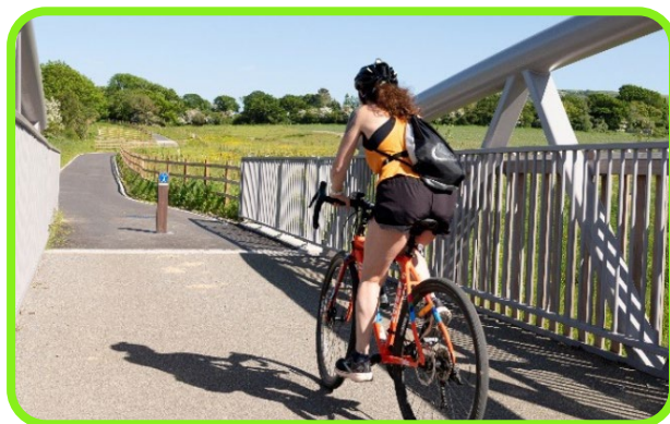
Figure 6-14: Bridge on the A27 active travel route which also provides for horse riders. See A27 East of Lewes case study.
