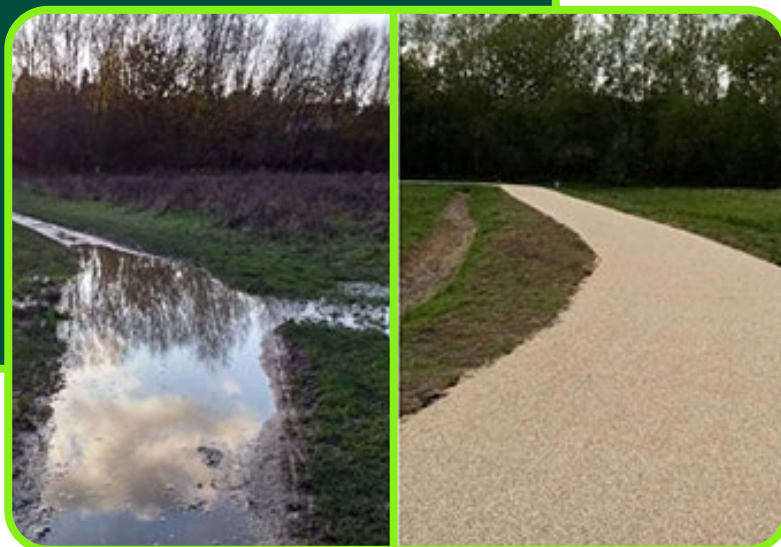
Figure 14-17: Path upgrade with new drainage system, Kennington Meadows, Oxfordshire.
