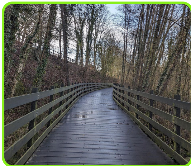
Figure 14-10: GRP boardwalk, Derbyshire.
