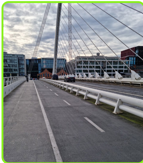
Figure 10-19: Flared parapets, Dublin.
