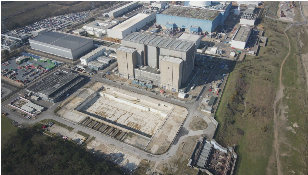
Image: Land now cleared where the Sizewell A turbine hall used to stand.
