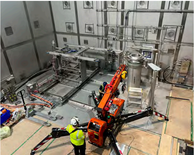
Machining Station Following Installation in the Process Cell.
