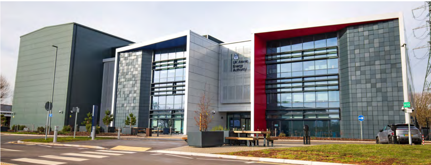
The UK Atomic Energy Authority in Culham where the H3AT Tritium Loop will be constructed.
