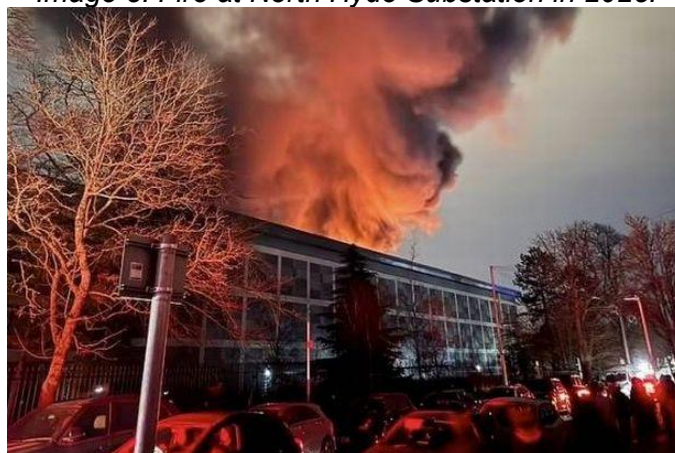
Image 8. Fire at North Hyde Substation in 2025.
