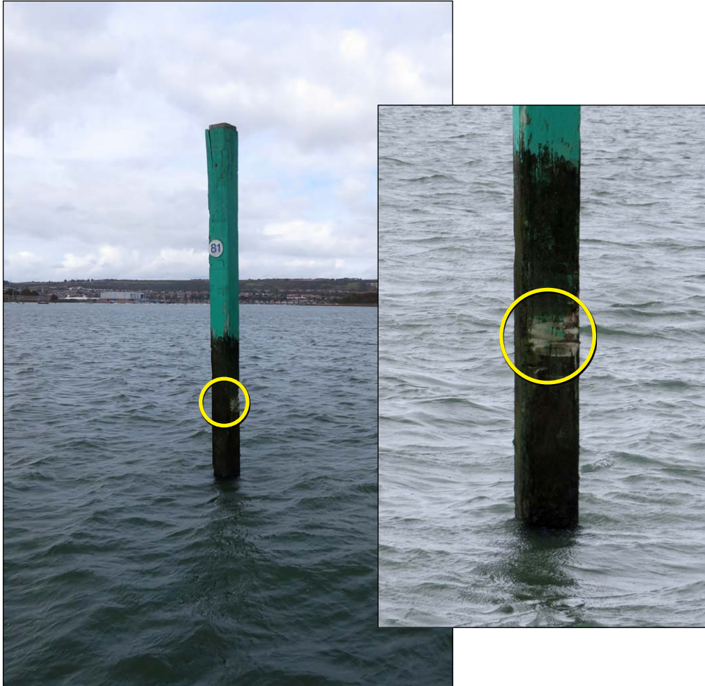
Figure 4: Navigation beacon 81 with inset detail of surface damage
