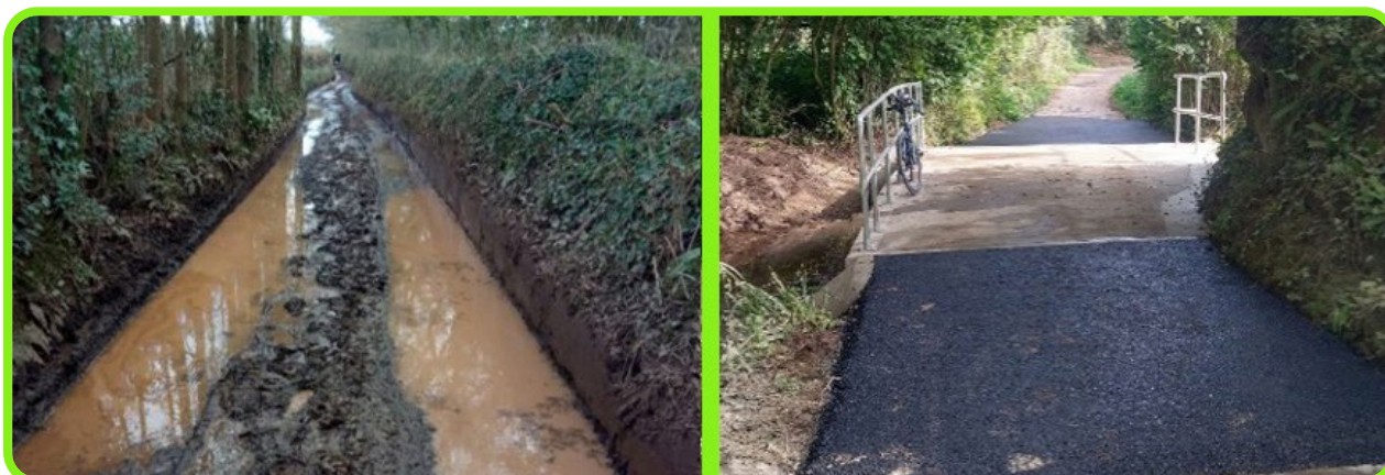
Figure 6: Rydon Lane before and after resurfacing.
