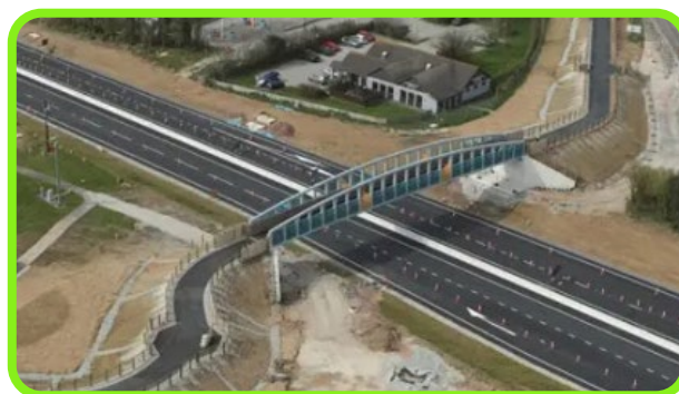
Figure 1: Chiverton Bridge, providing an active travel link over the A30.
