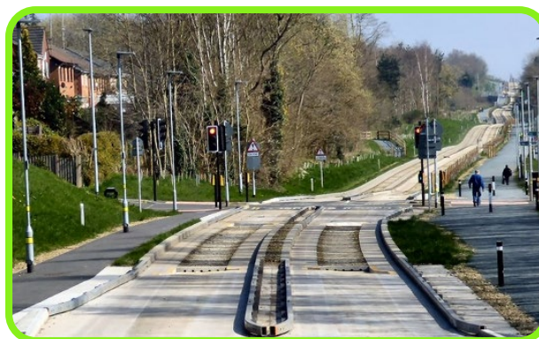
Figure 3: Controlled crossing at Well Street junction with busway.
