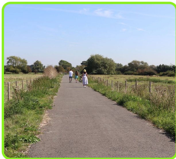
Figure 1: St Peter's Greenway provides a year-round facility for leisure and utility journeys.
