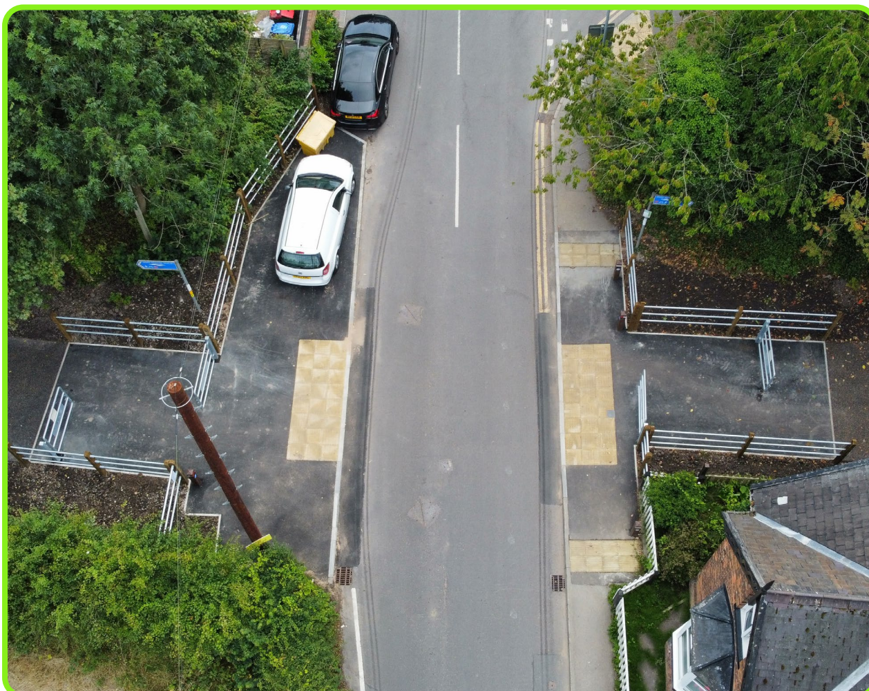
Figure 9: Completed section of the Trans Pennine Trail.
