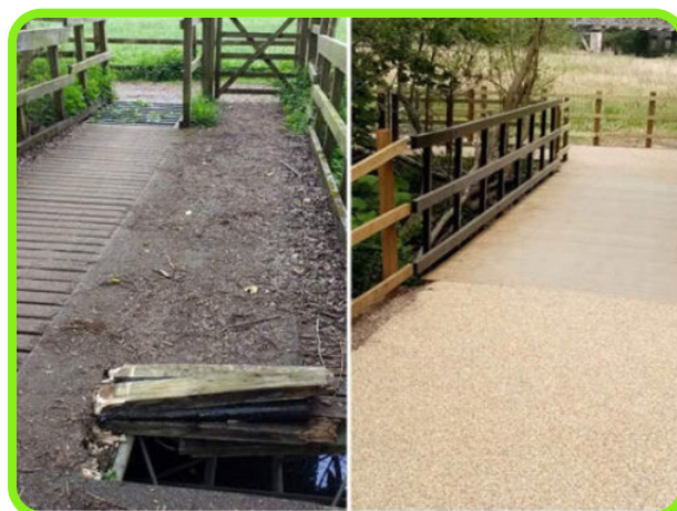
Figure 5: Before and after showing renewed bridge.
