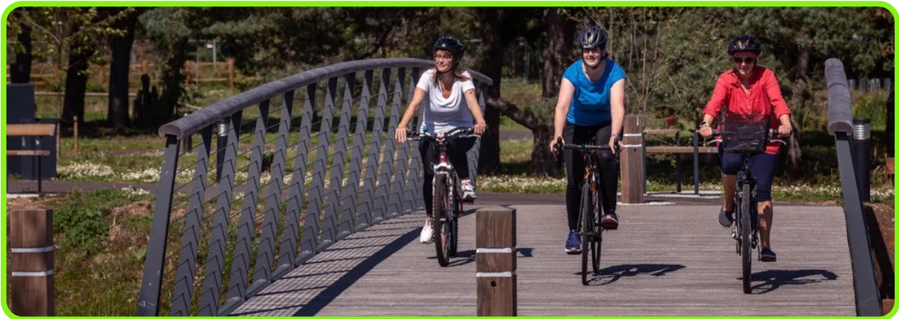
Figure 6: A completed section of Waterbeach with active travel provision.
