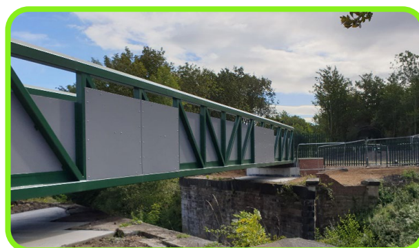
Figure 5: Newly constructed bridge across the railway.
