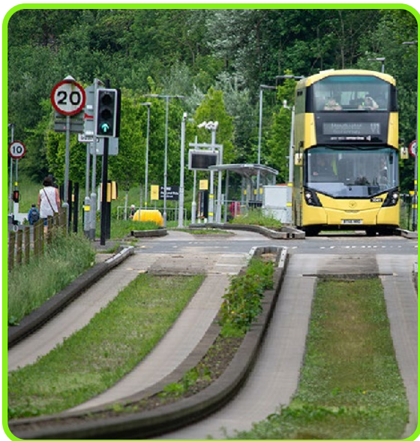
Figure 5: Signalised junction enabling easy access for pedestrians and cyclists.
