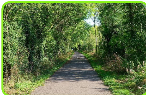
Figure 10: Completed section of the Lias Line.
