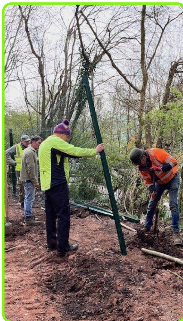
Figure 11: Fencing being installed by Strawberry Line volunteers.
