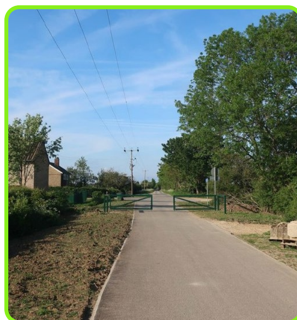
Figure 9: Completed resurfacing on Mere Way.
