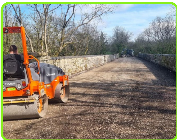
Figure 4: Hamwood viaduct, Somerset Circle.
