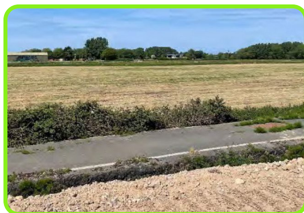
Figure 7: Wild Lane prior to resurfacing and upgrade.
