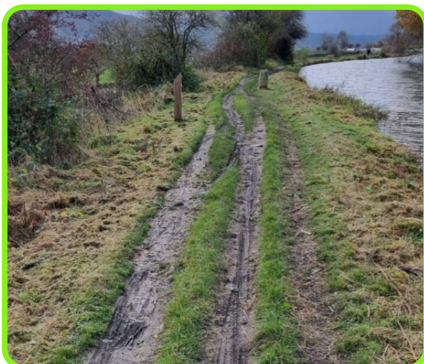
Figure 3: View of towpath before and after improvement works.
