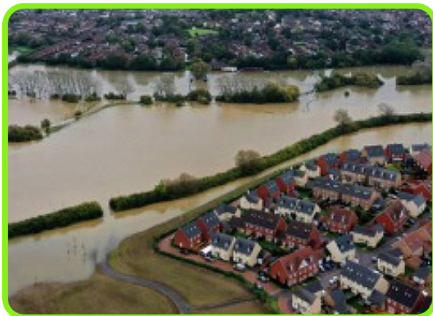
Figure 5: Flooding in Buckingham Park.
