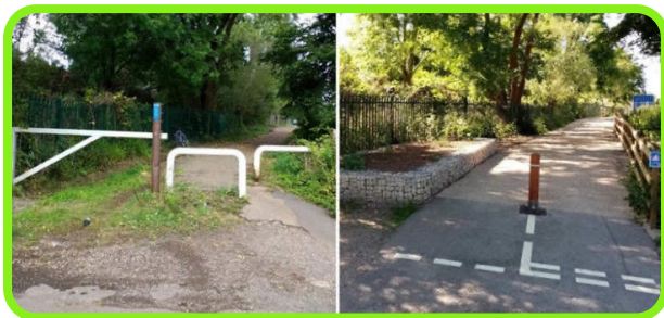
Figure 7: Before and after showing improved access at Sandford Lane.
