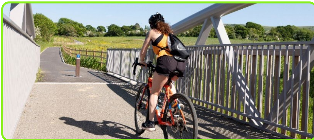
Figure 5: New bridge structures were required to enable the route.
