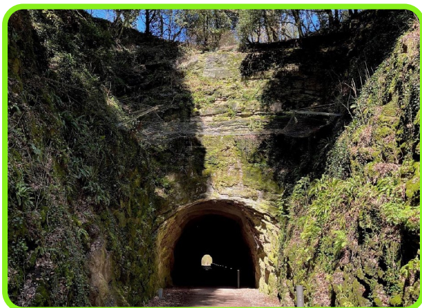
Figure 7: Shute Shelve Hill Tunnel.
