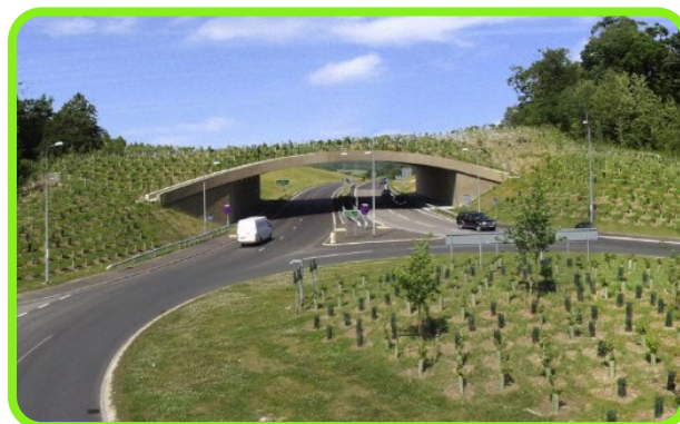
Figure 10-15: Scotney Castle Land Bridge, Kent.
