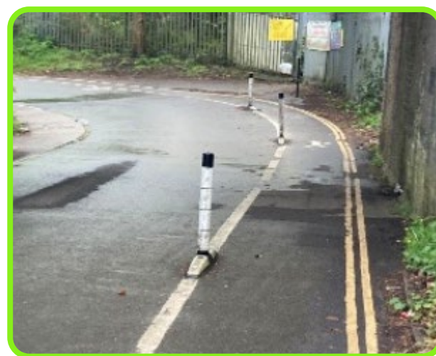
Figure 7-16: Implied footway protected by wands, Surrey.
