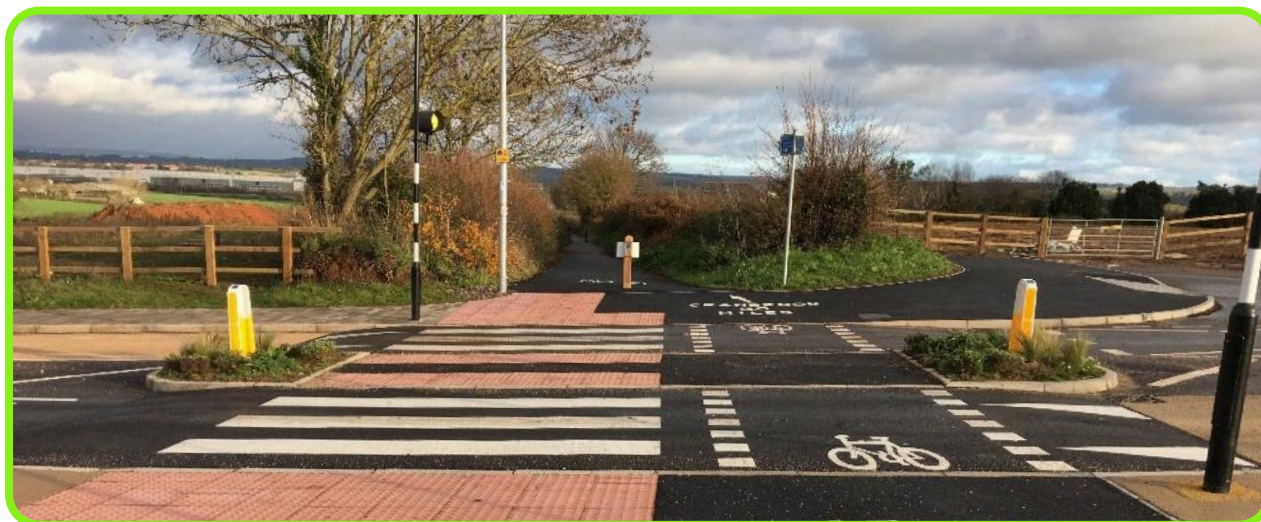
Figure 13-8: Blackhorse Lane, Exeter was stopped up to vehicle traffic when the new Tithebarn Link Road was constructed, including a parallel crossing on the desire line to cross it.
