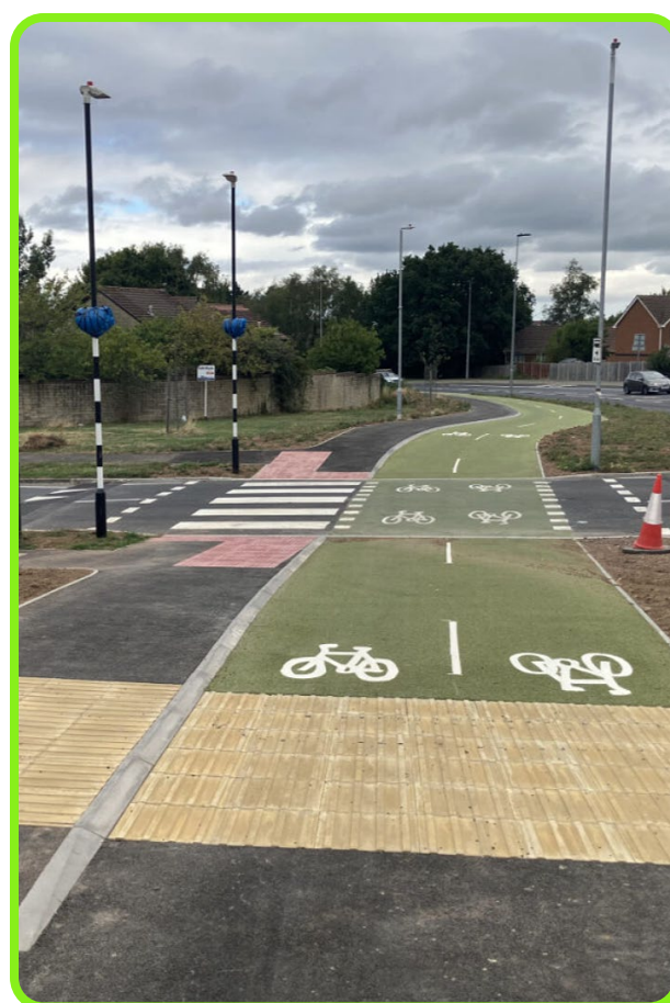
Figure 10-20: Off-carriageway route crossing minor road, South Gloucestershire.
