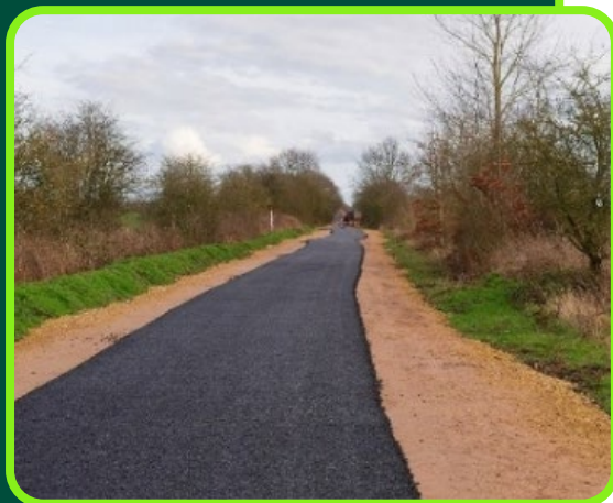
Figure 14-5: Newly installed asphalt on the Lias Line, with trotting strip provided either side.
