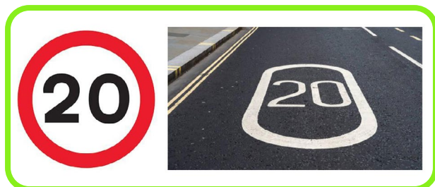
Figure 12-7: Speed limit signs: upright sign to diagram 670 and road sign to diagram 1065.
