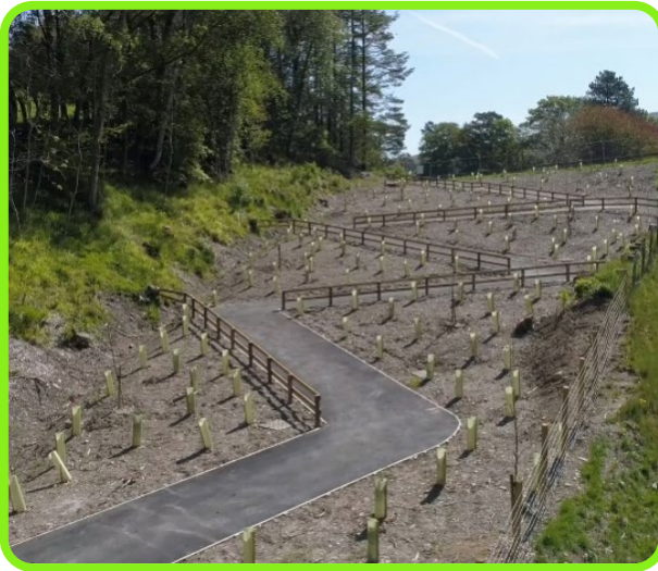
Figure 5-5: Zig-zag path, shortly after construction, to reduce steep gradient to A66. See Keswick to Threlkeld case study.
