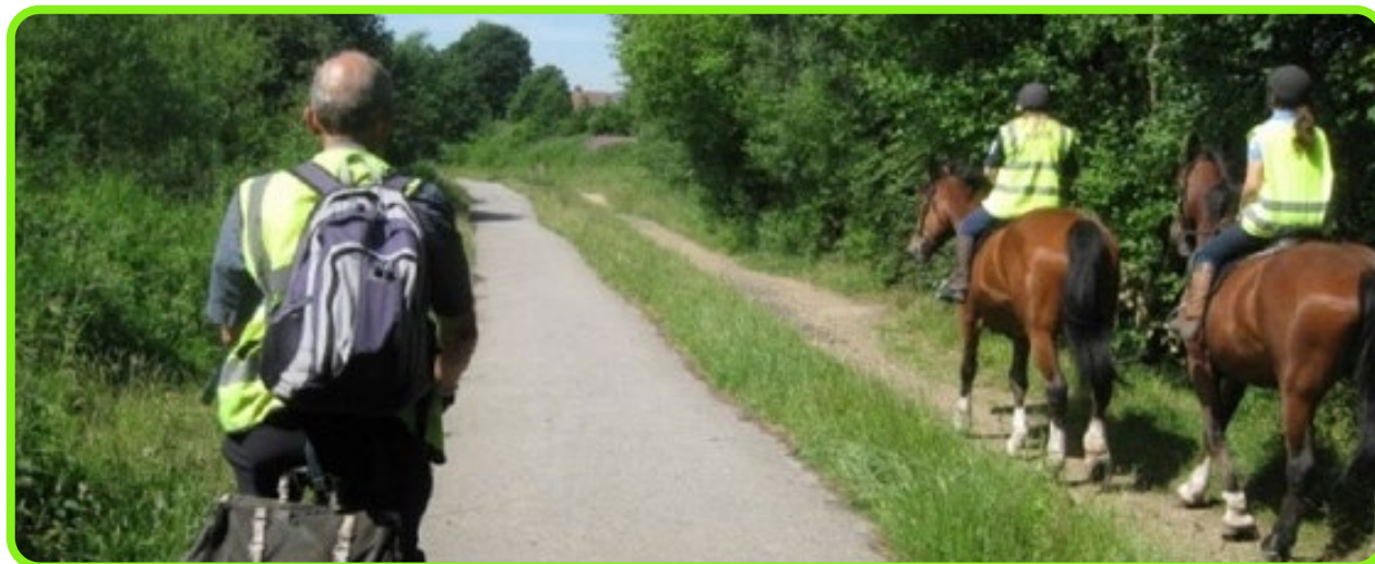
Figure 4-4: Trotting strip alongside a pedestrian/cycle path.
