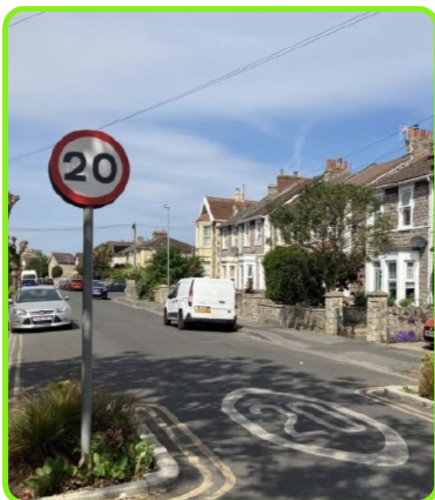
Figure 7-6: Gateway with signing and narrowing, North Somerset.
