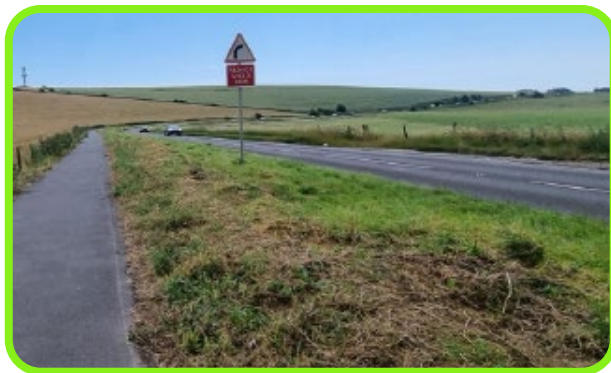
Figure 6-6: Separation of active travel route by distance, noise bank and planting.
