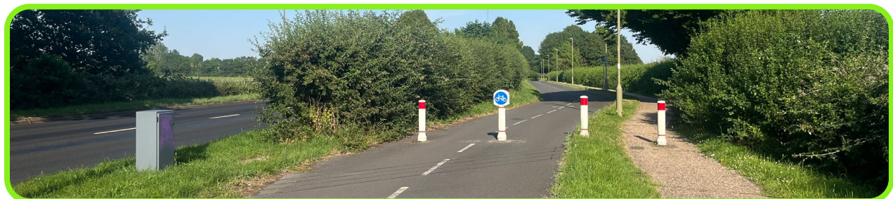
Figure 6-7: Separation of active travel route by distance, noise bank and planting.
