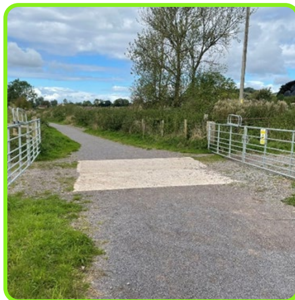
Figure 8-28: Concrete crossing pad and gates.
