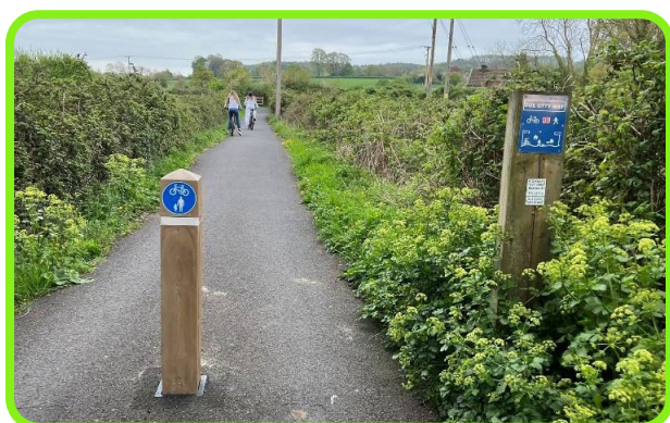
Figure 8-22: Single bollard arrangement – Flax Bourton, North Somerset.
