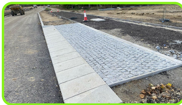
Figure 14-13: Precast concrete edge, Coalville.
