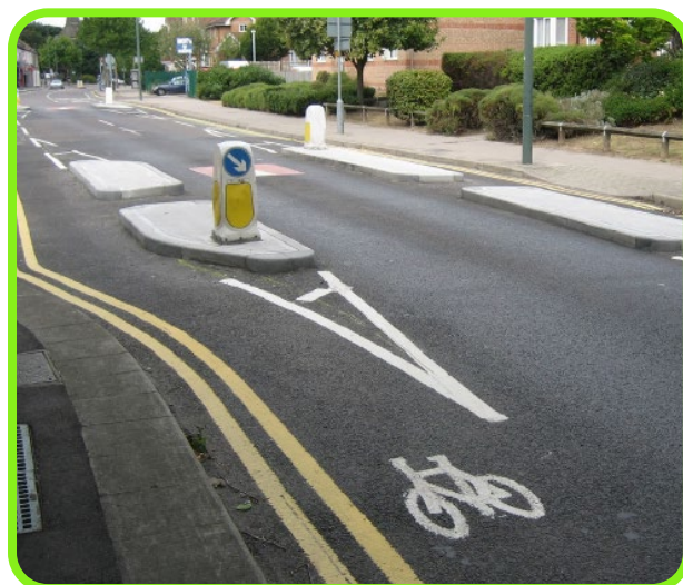
Figure 6-11: Single lane narrowing with advisory cycle lanes, London.
