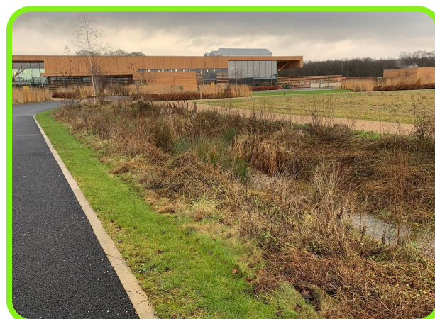
Figure 14-15: Swale between vehicle access route and shared path – RHS Bridgewater.
