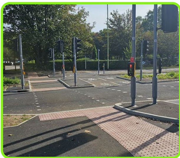
Figure 10-7: Parallel, separated pedestrian and cycle crossing, Hampshire.
