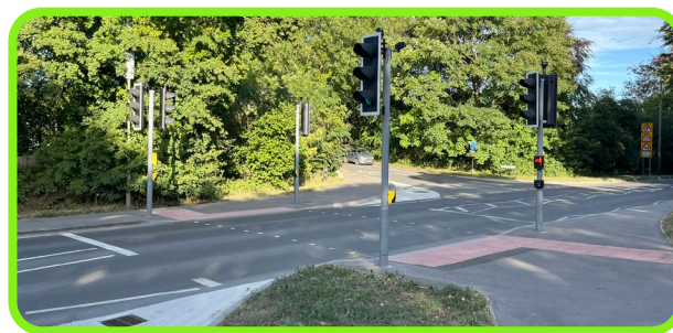
Figure 10-11: Signal-controlled crossing linking Chilton Road and Station Road across A417, Oxfordshire.
