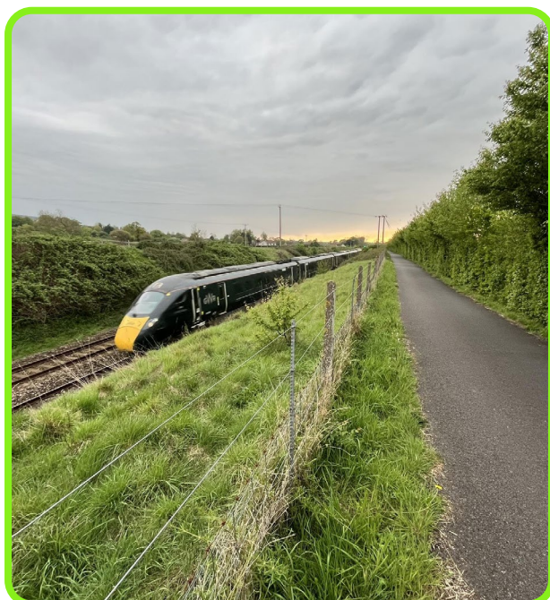
Figure 8-10: Path adjacent to the Bristol to Exeter line as it passes through North Somerset.
