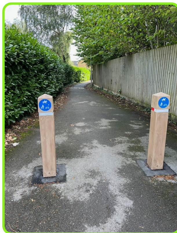
Figure 8-23: Double bollard arrangement – Nailsea, North Somerset.
